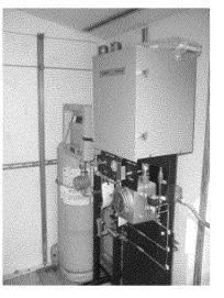
The 4<sup>th</sup> step is SoCalGas installs appropriate GC, carbon dioxide, oxygen, moisture, and hydrogen sulfide continuous monitors downstream of the conditioned biogas production point for direct monitoring and control.
