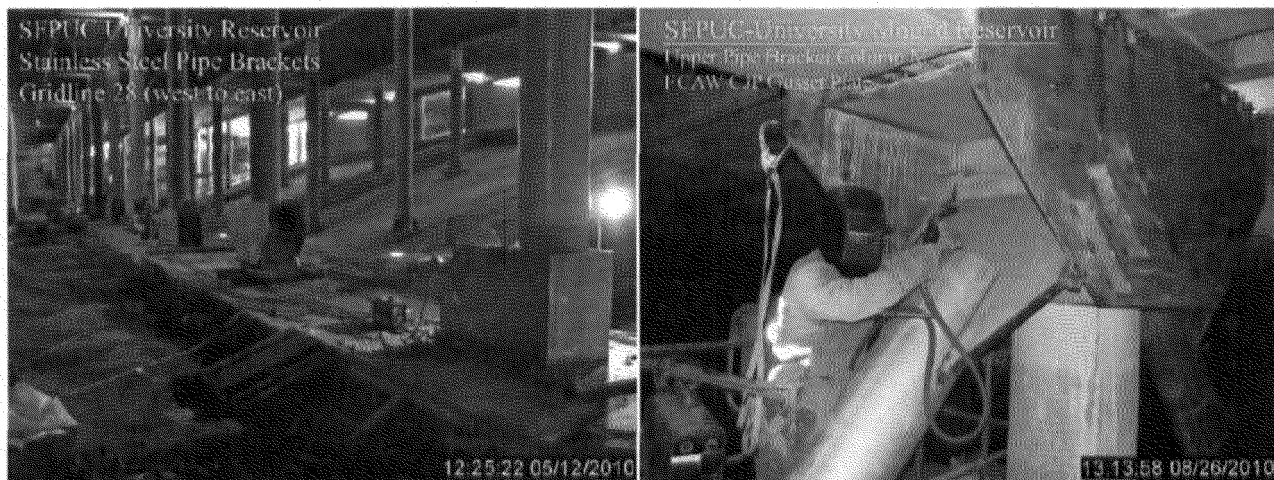
View of the interior of the Reservoir during the retrofit.
