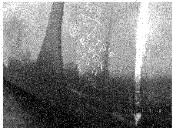
Final inspection, CJP on 14" wide backing strap
