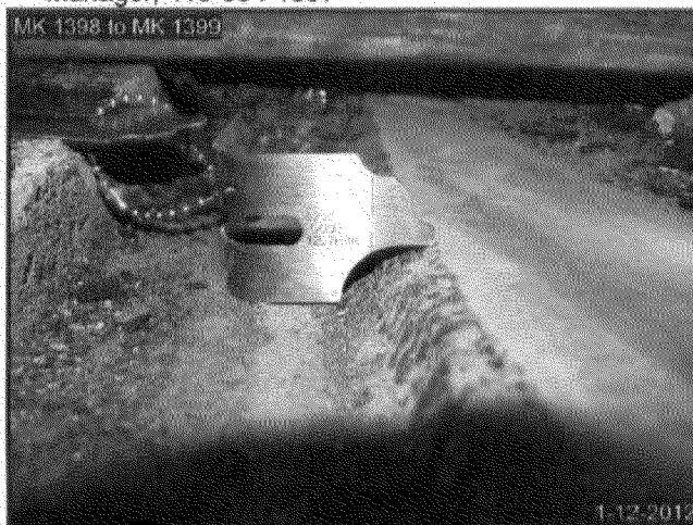
Measurement of interior and exterior fillet welds.
