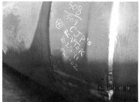
Final inspection, CJP on 14" wide backing strap
