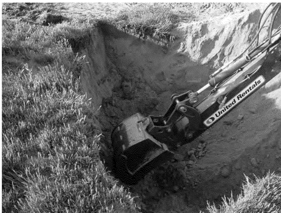
Photo 8. Reaching final depth of approximately 9 feet below ground surface at location 2. Looking northwest. March 12, 2013.
