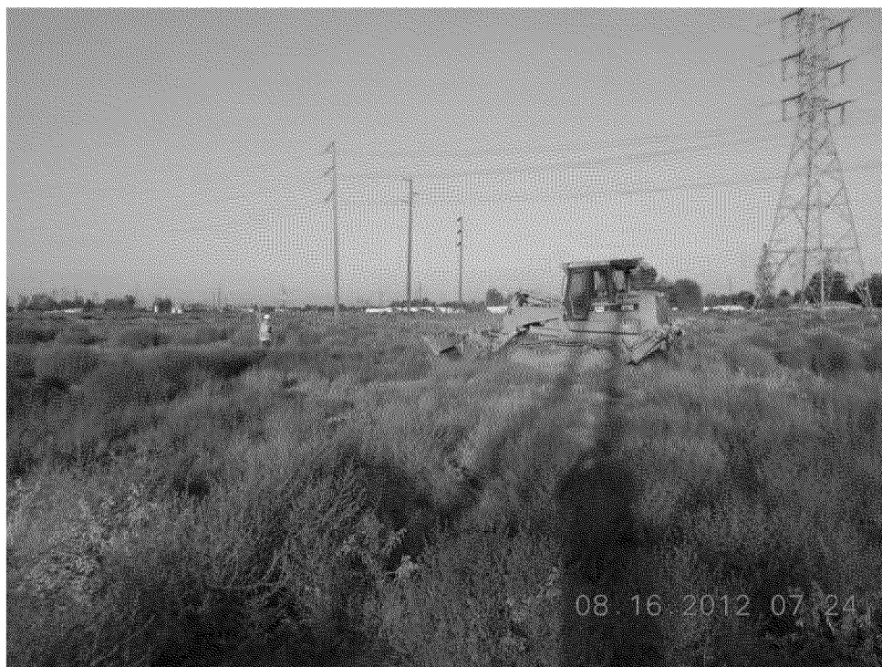
Photo 2. Attempting to locate WS7. Looking southwest. August 16, 2012.
