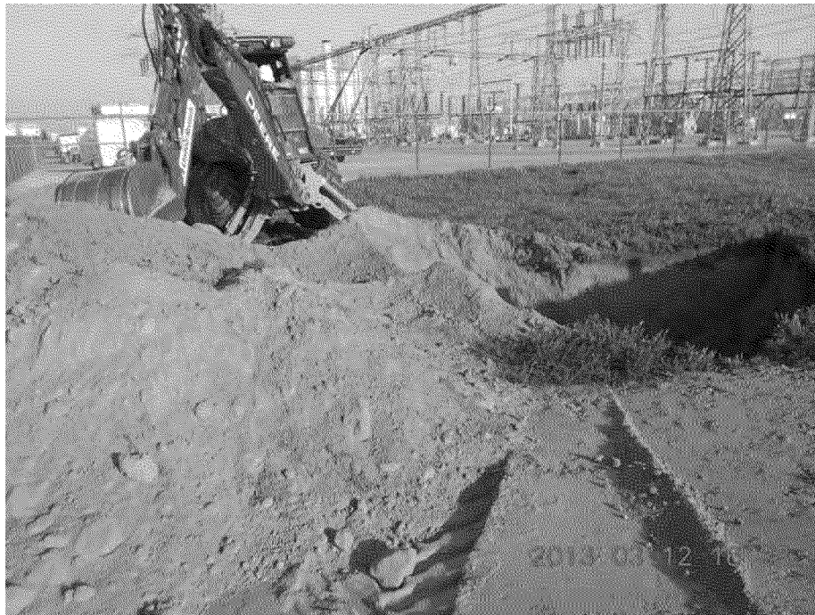
Photo 7. Excavation of location 2 for WS5. Looking southeast. March 12, 2013.
