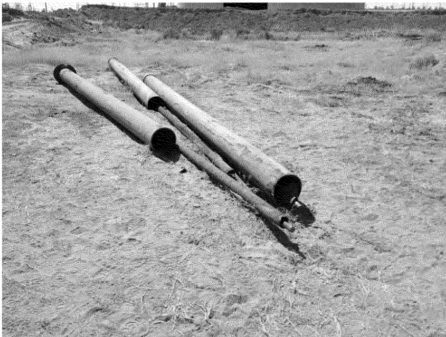
Photo 14. Sixty feet of pump casing removed from WS1. Looking west. April 18, 2013.
