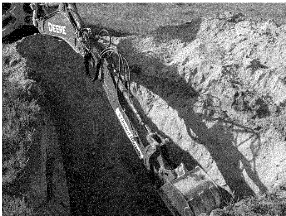
Photo 6. Reaching final depth of approximately 8 feet below ground surface in location 1. Looking northwest. March 12, 2013.
