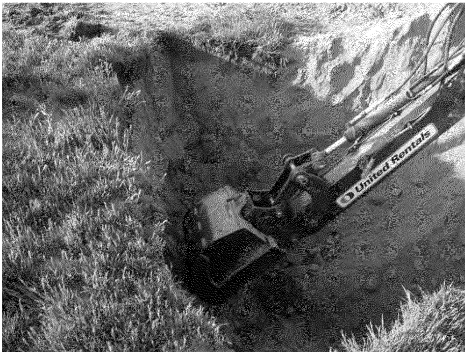
Photo 8. Reaching final depth of approximately 9 feet below ground surface at location 2. Looking northwest. March 12, 2013.
