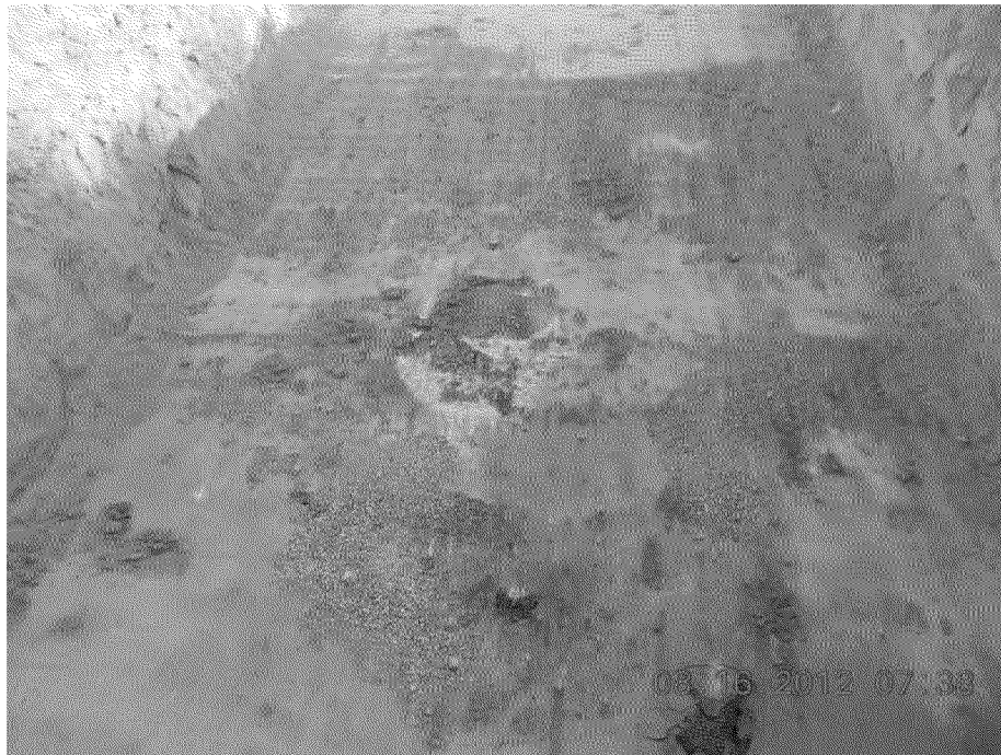
Photo 3. Cement grout found approximately 5 feet below ground surface at WS7 search area. Looking north. August 16, 2012.
