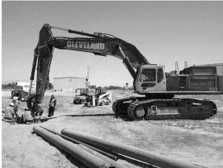
Photo 13. Removed pump casing and driveshaft from WS1. Attempting to free remaining pump from the well. Looking east. April 18, 2013.
