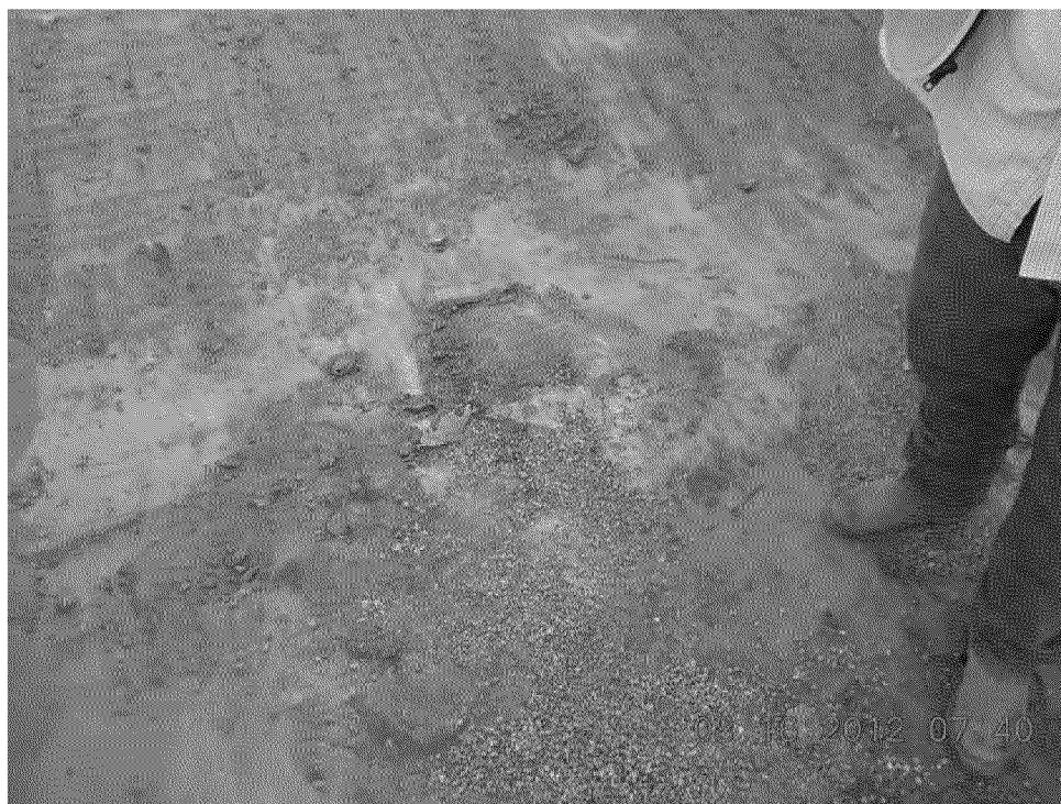
Photo 4. Cement grout seal of WS7. Looking north. August 16, 2012.
