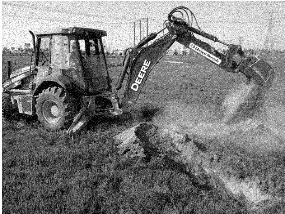
Photo 5. Beginning excavation to find WS5 at location 1. Looking northwest. March 12, 2013.
