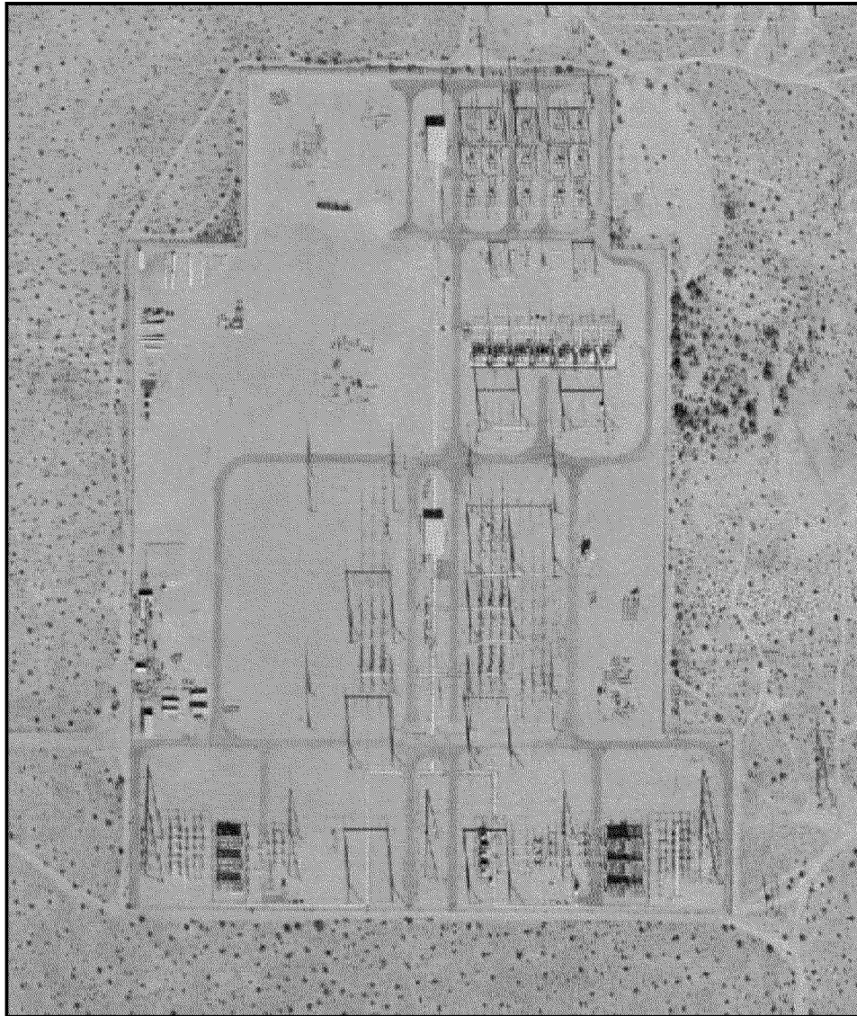
Figure 3: Imperial Valley substation
