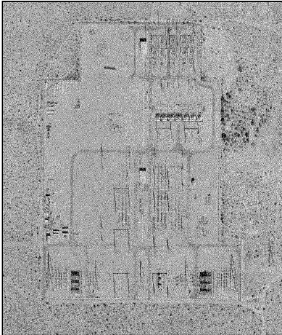
Figure 3: Imperial Valley substation
