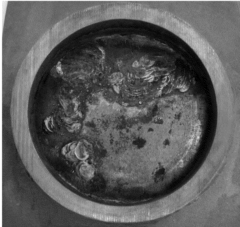
(a) Photograph of area under PLIDCO cap after cleaning
