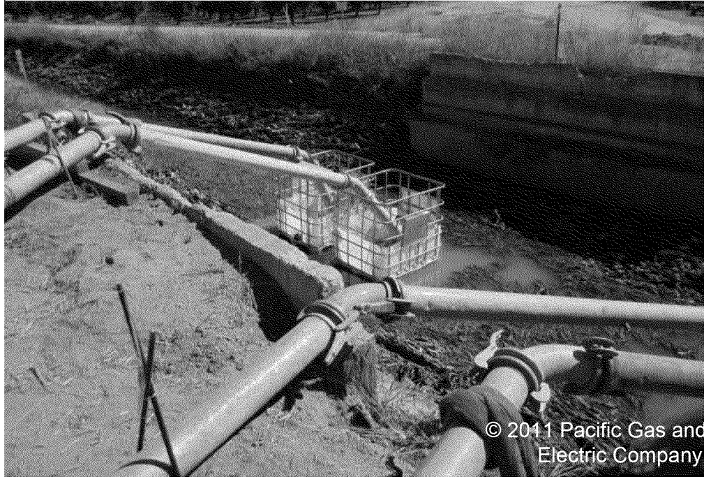
Water disposal in a drainage/irrigation canal
