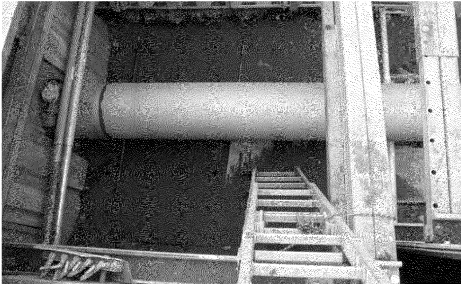
Overview of clean blasted inspection area prior to recoat activities
