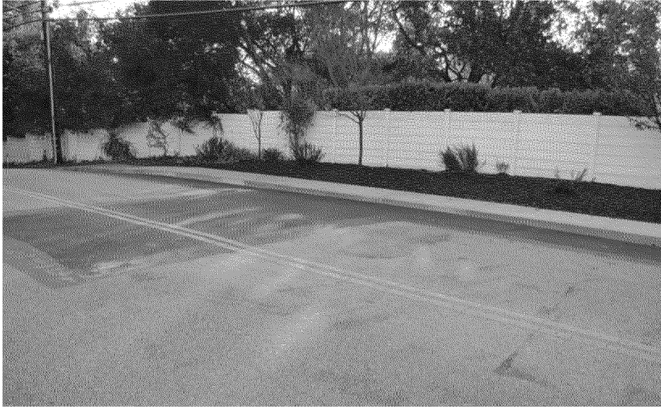
Overview of completed Cover looking upstream
