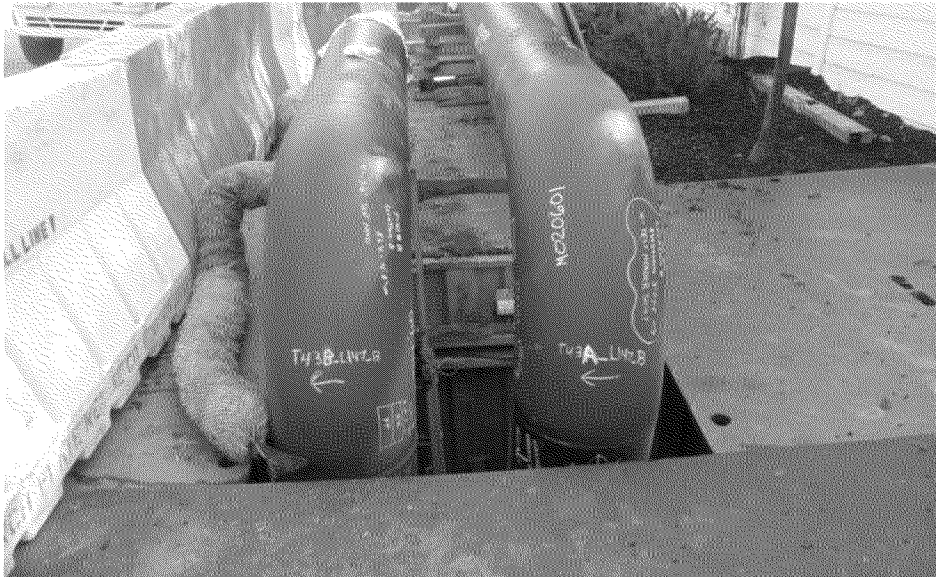
Overview of T43A(US) & T43B(DS) in same excavation.
