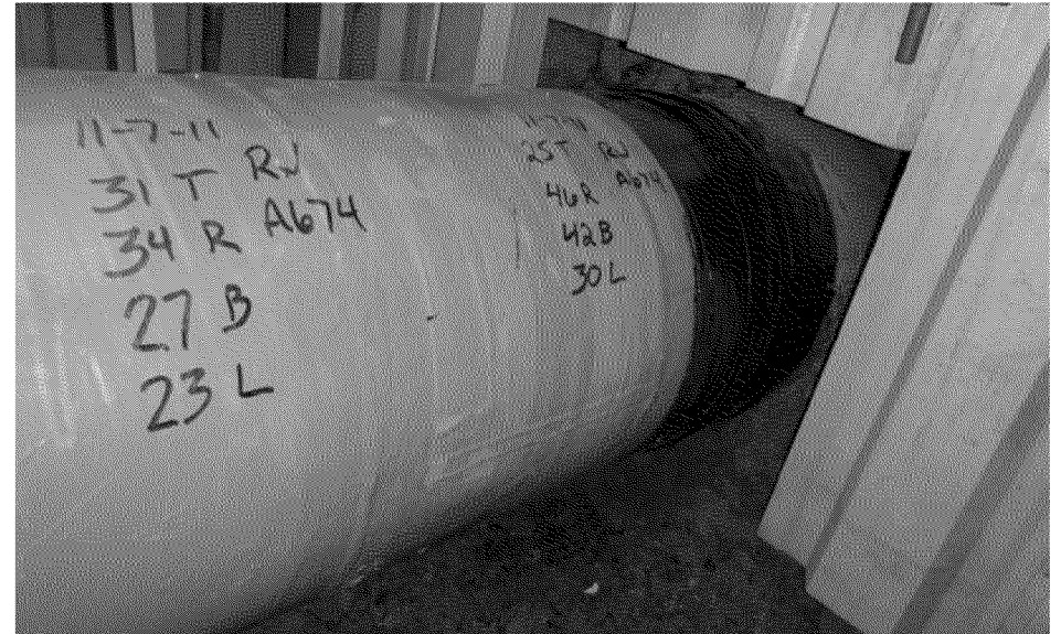
Overview of final coating condition US 3:00
