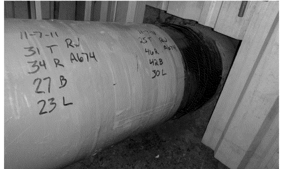
Overview of final coating condition US 3:00
