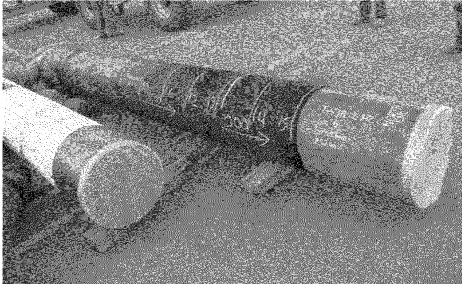
Removed pipe section coating assesment 3:00
