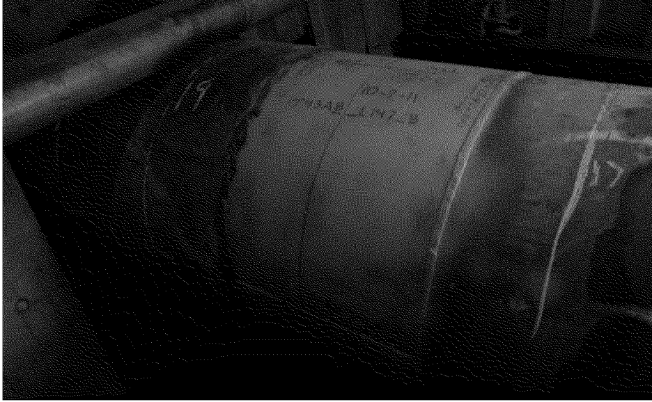
Overview of coating condition 17ft to 20ft, 9:00 position
