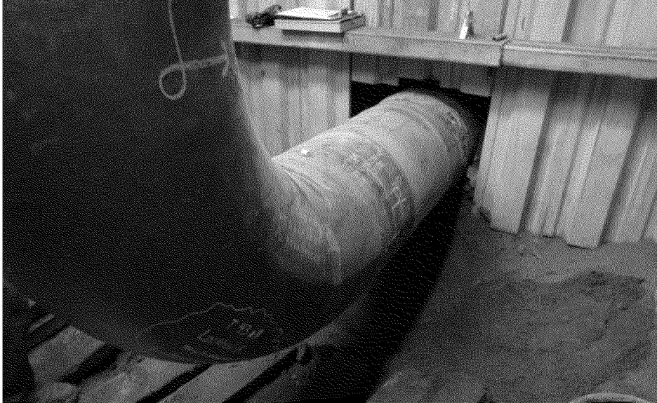
Overview of coating condition -1ft to 2ft, 9:00 position
