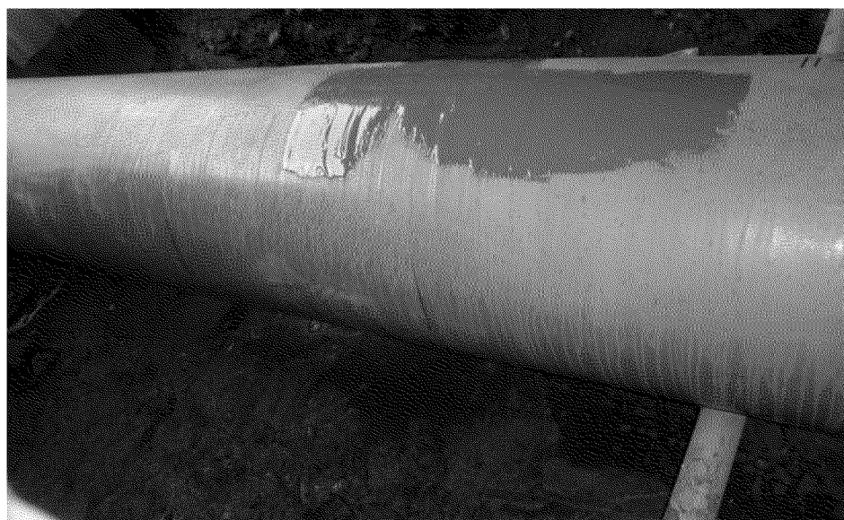
Overview of final coating condition 3:00
