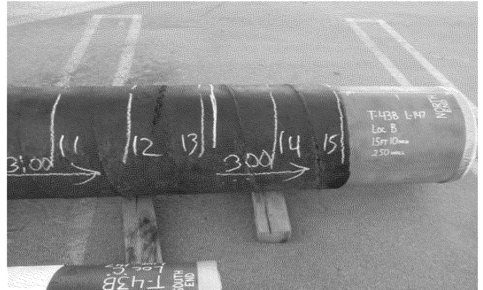
Overview of coating condition 3:00 position
