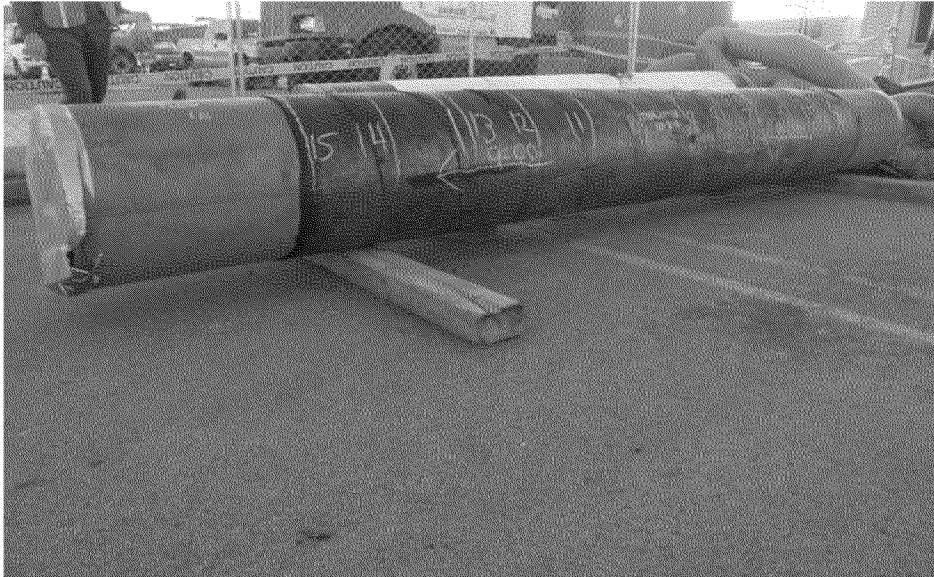
Removed pipe section coating assesment 9:00
