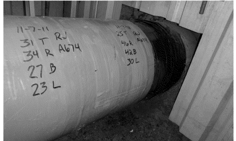
Overview of final coating condition US 3:00
