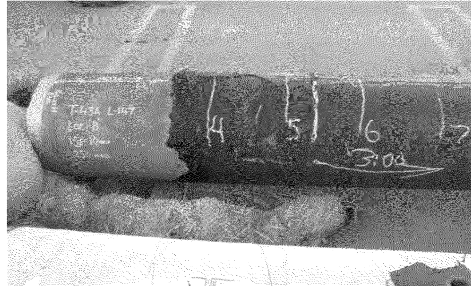
Overview of coating condition 3:00 position
