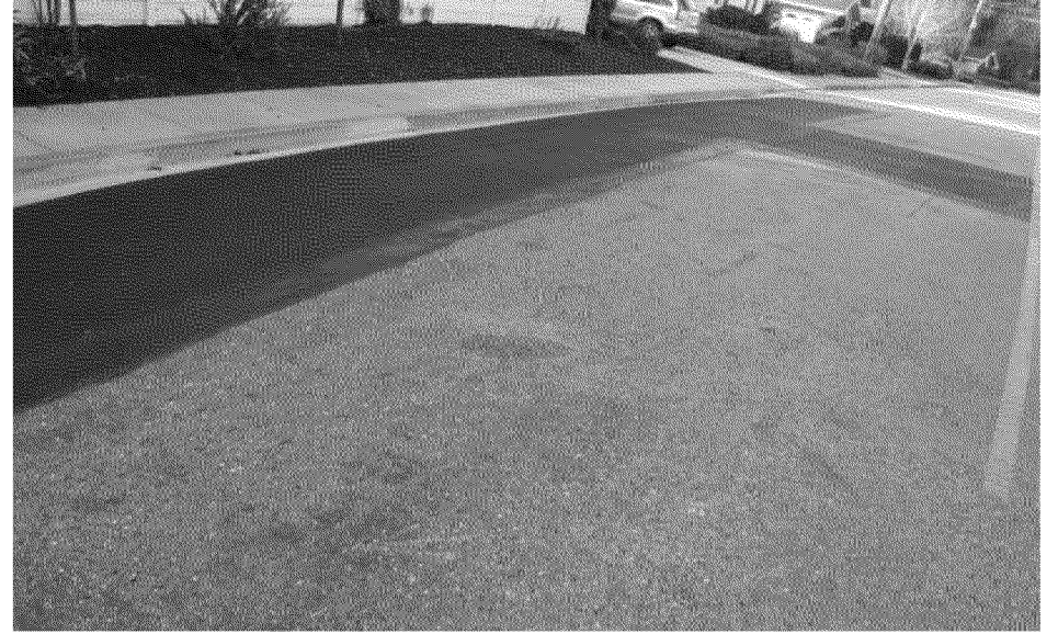
Overview of completed Cover, 9:00 view
