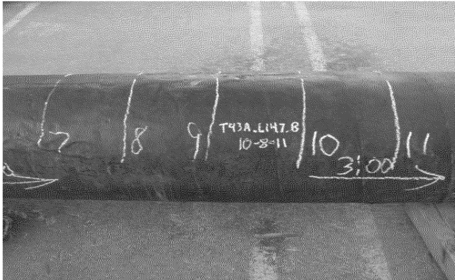
Overview of coating condition 3:00 position
