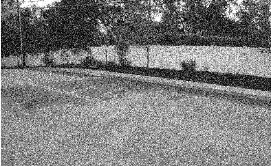
Overview of completed Cover looking upstream
