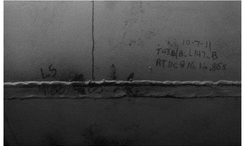
Overview of feature joint long seam @ 8:55
