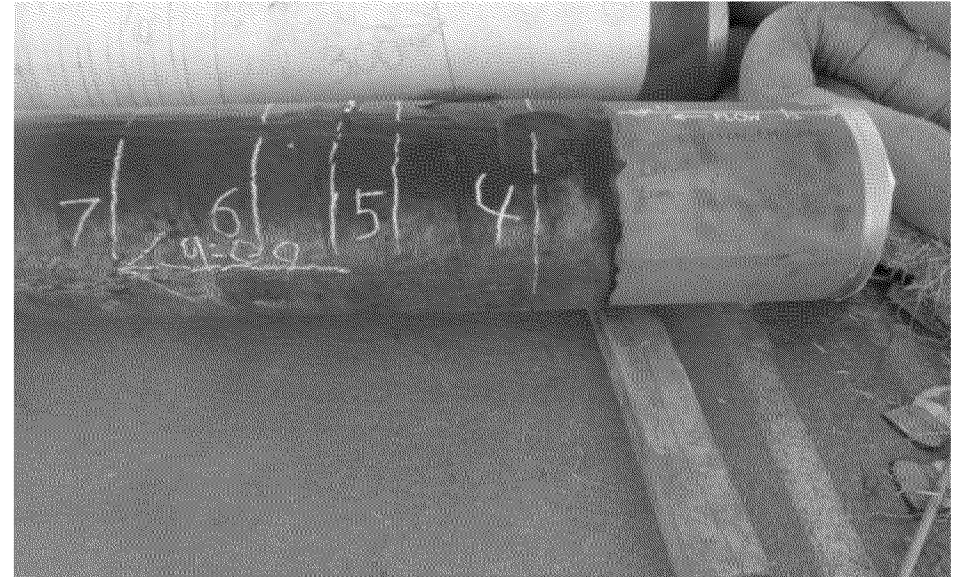
Overview of coating condition 9:00 position
