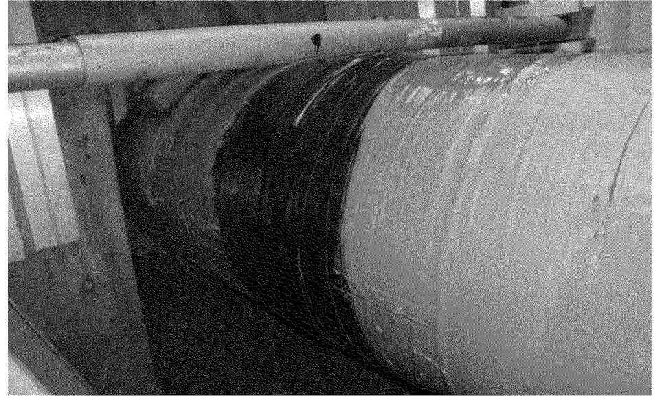
Overview of final coating condition US 3:00
