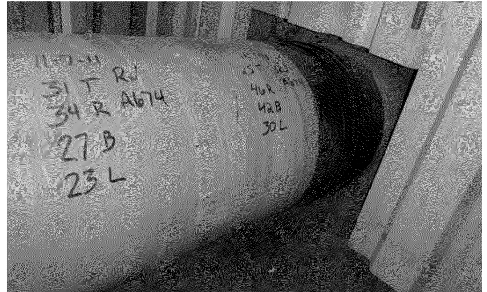
Overview of final coating condition US 3:00
