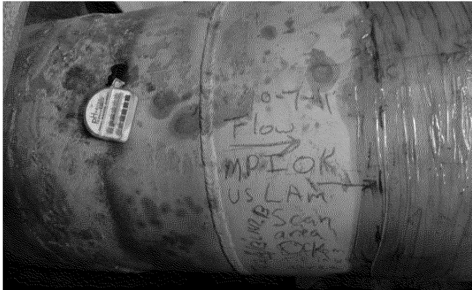
Overview of pipe Ph.
