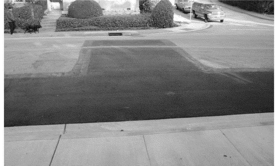
Overview of completed Cover looking downstream
