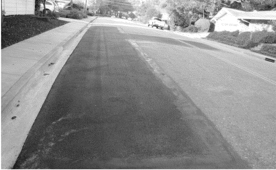
Overview of completed Cover, 3:00 view
