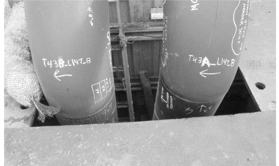
Closeup of T43A(US) & T43B(DS) in same excavation.
