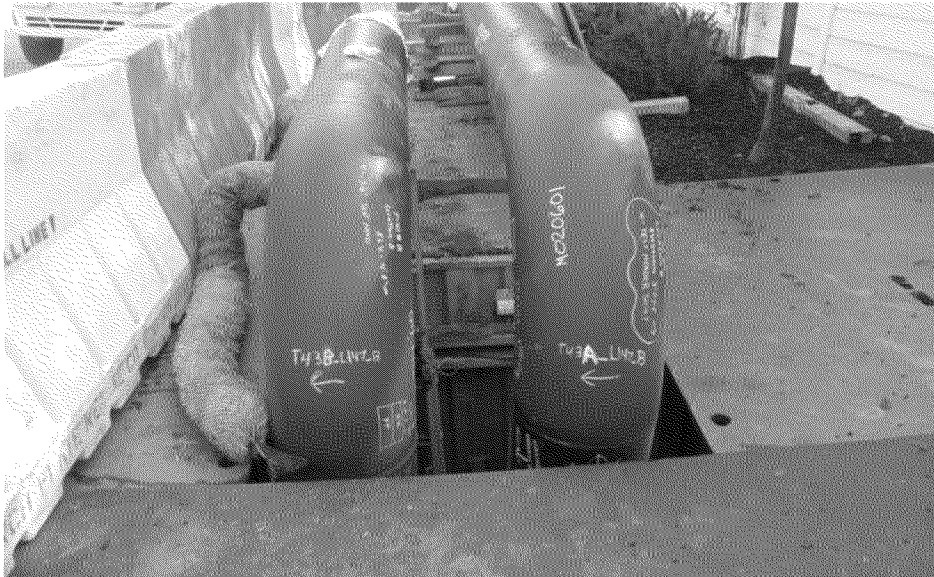
Overview of T43A(US) & T43B(DS) in same excavation.
