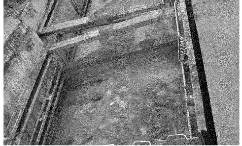
Overview of completed Slurry
