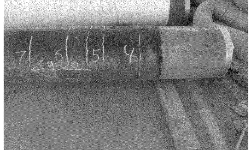
Overview of coating condition 9:00 position
