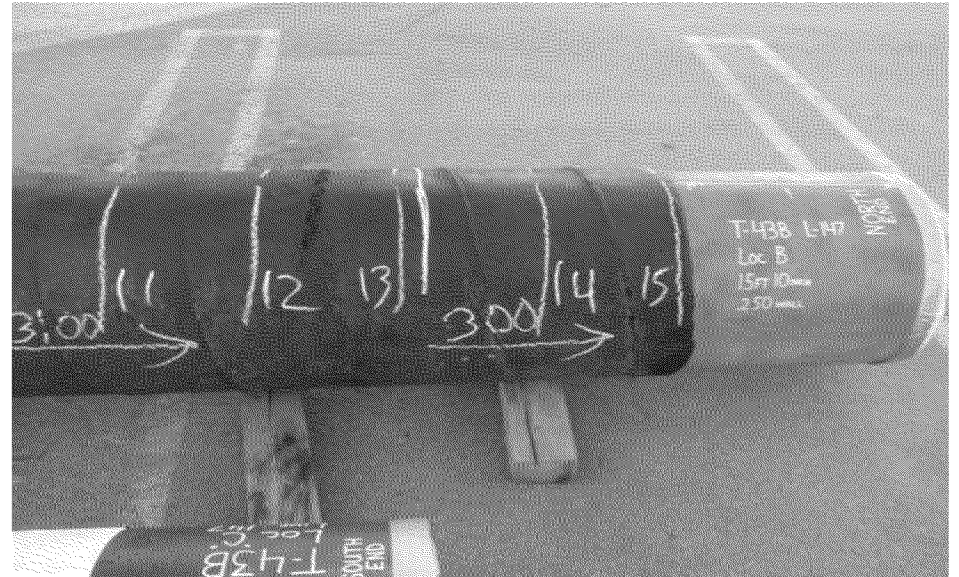
Overview of coating condition 3:00 position
