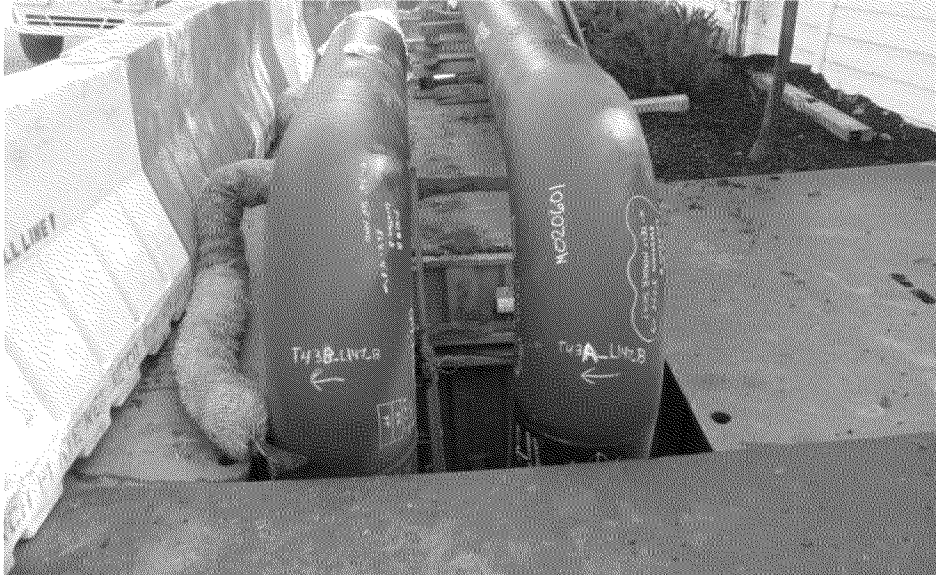
Overview of T43A(US) & T43B(DS) in same excavation.
