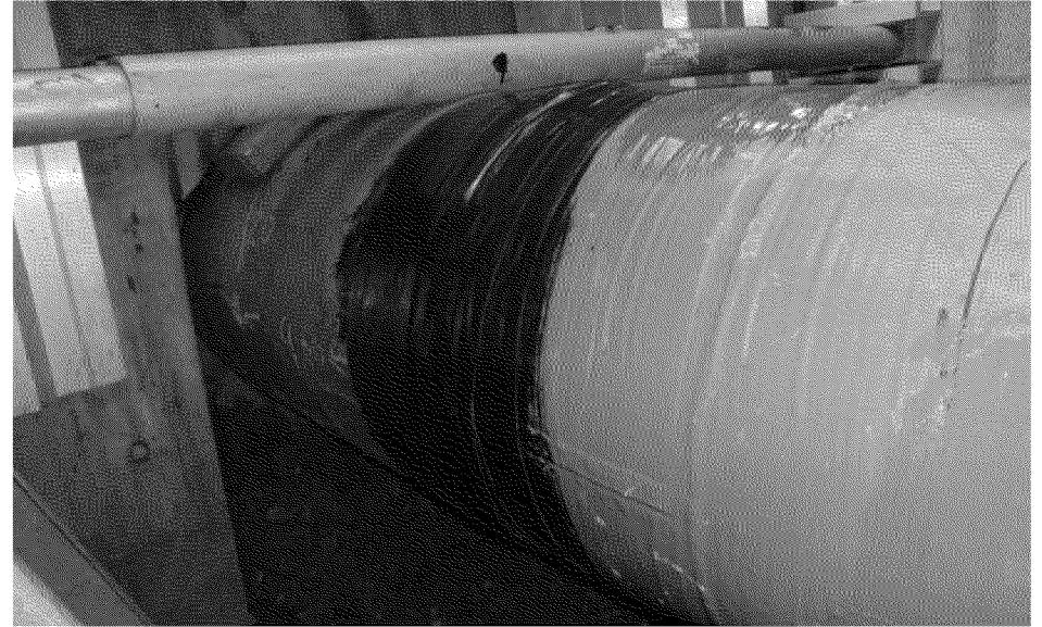
Overview of final coating condition US 3:00
