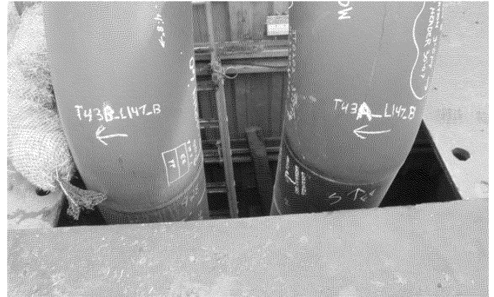
Closeup of T43A(US) & T43B(DS) in same excavation.
