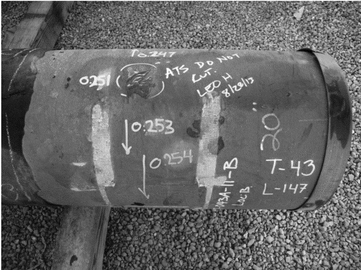
Downstream end of spool
