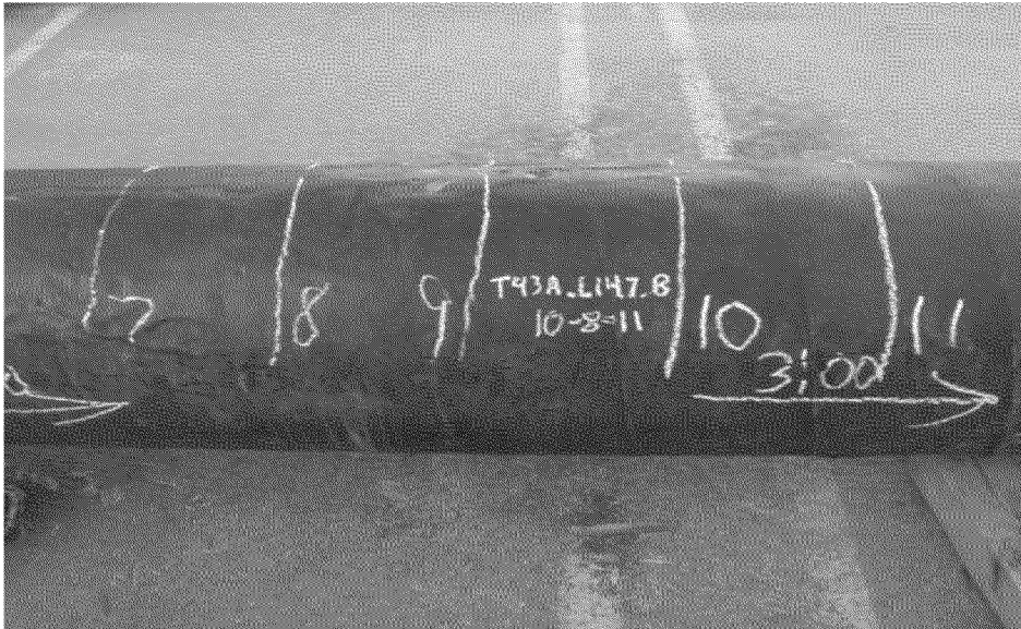
Overview of coating condition 3:00 position
