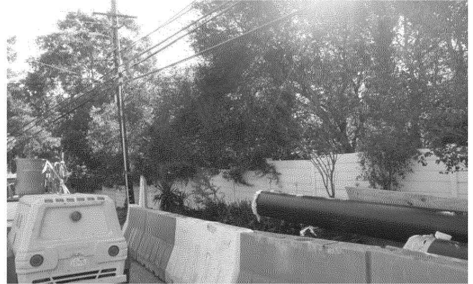
Typical surrounding topography
