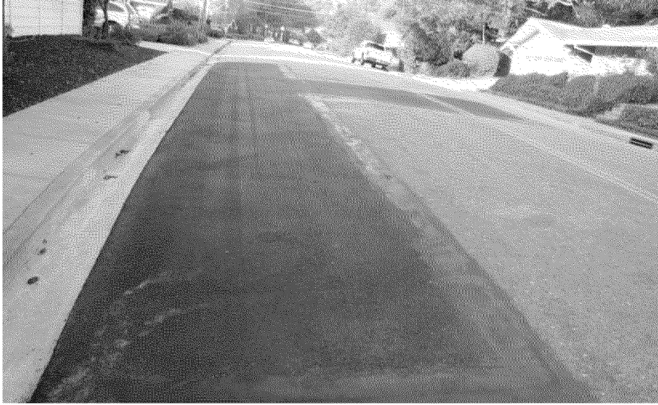
Overview of completed Cover, 3:00 view
