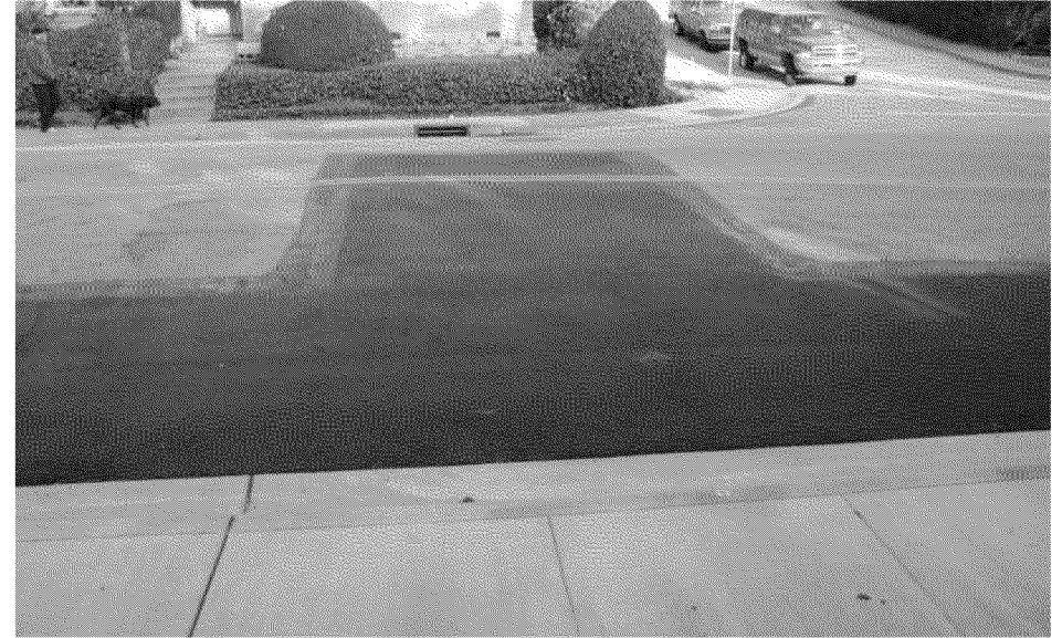
Overview of completed Cover looking downstream
