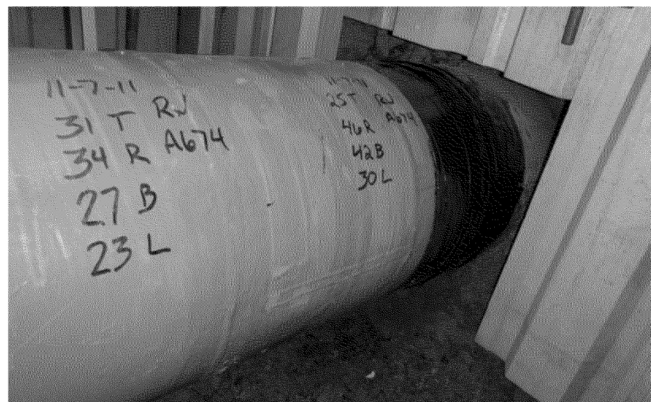
Overview of final coating condition US 3:00
