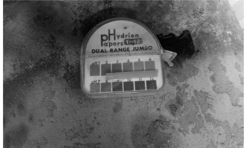
Closeup of pipe Ph.
