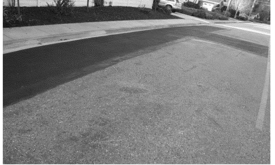
Overview of completed Cover, 9:00 view
