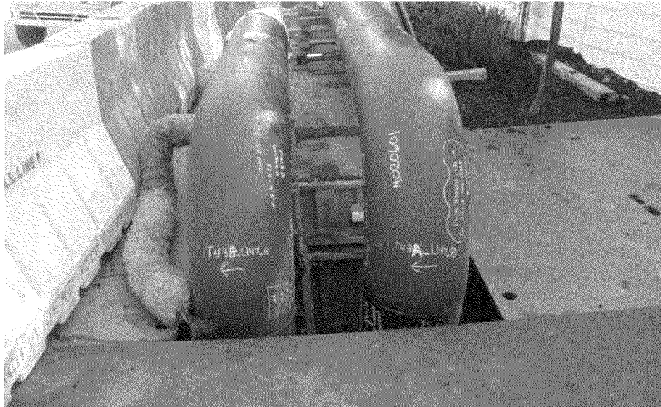
Overview of T43A(US) & T43B(DS) in same excavation.
