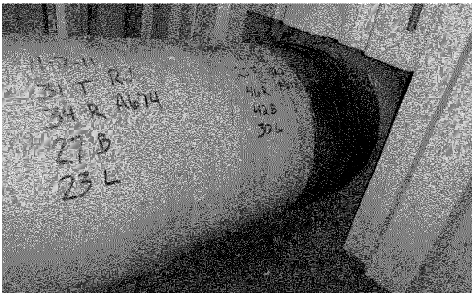
Overview of final coating condition US 3:00
