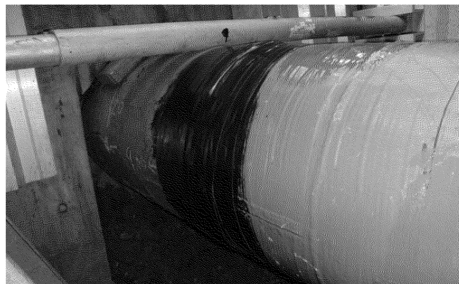
Overview of final coating condition US 3:00
