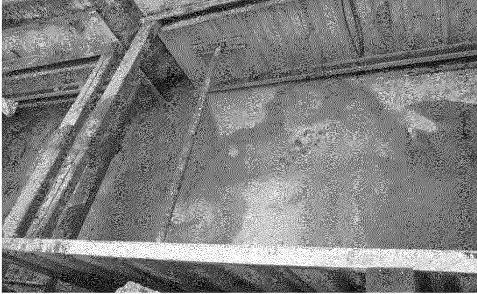
Overview of completed Slurry
