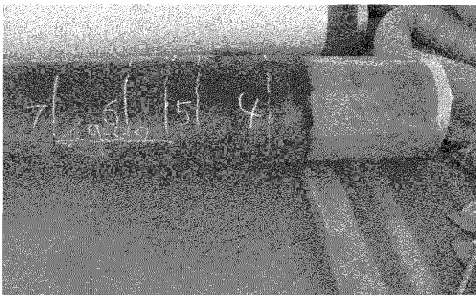
Overview of coating condition 9:00 position
