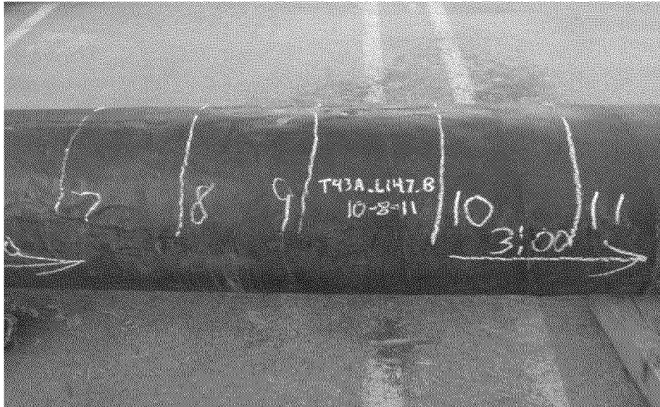
Overview of coating condition 3:00 position
