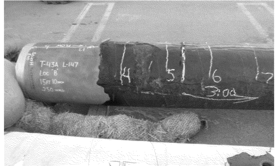
Overview of coating condition 3:00 position
