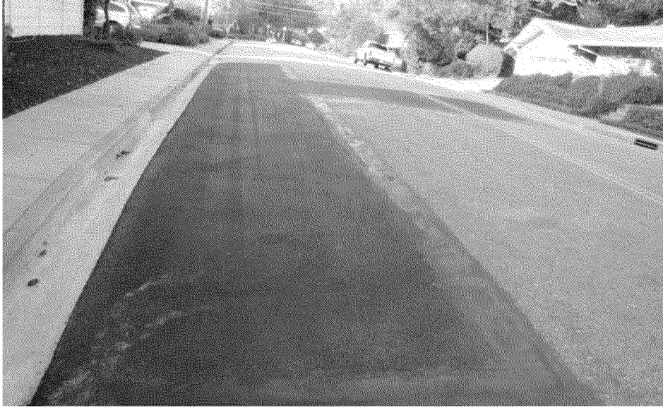
Overview of completed Cover, 3:00 view
