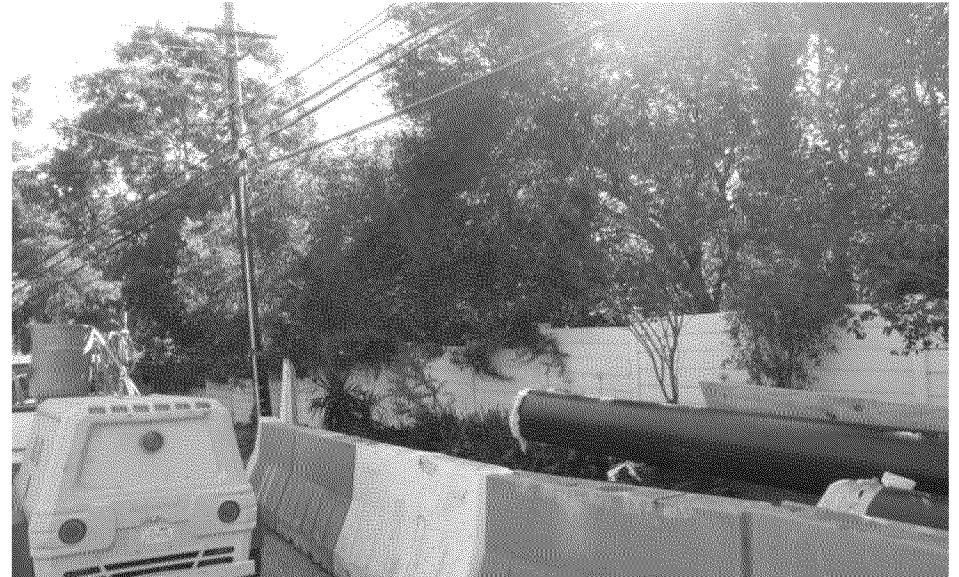
Typical surrounding topography
