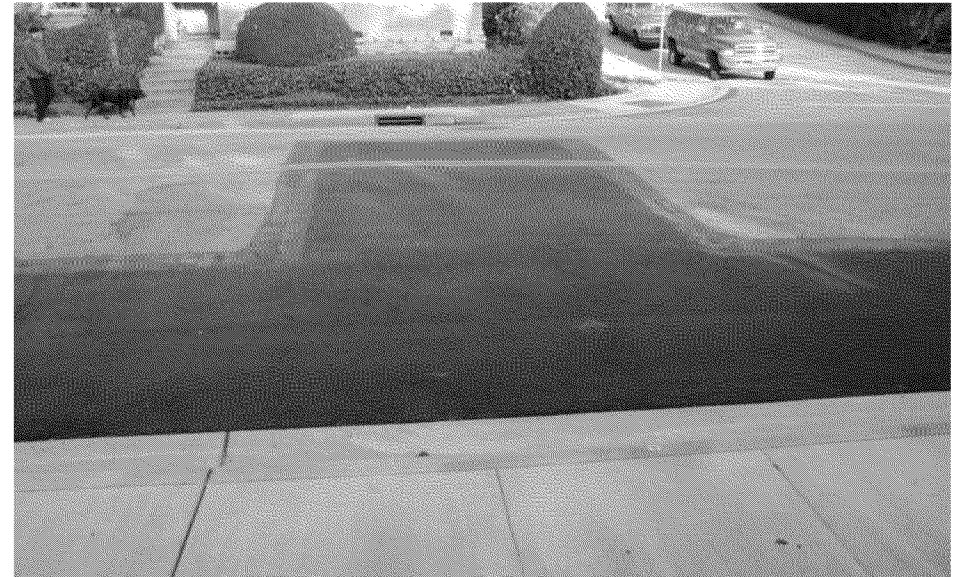
Overview of completed Cover looking downstream
