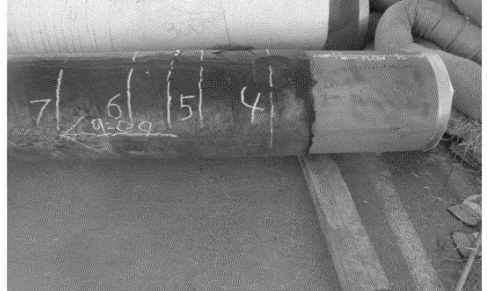
Overview of coating condition 9:00 position
