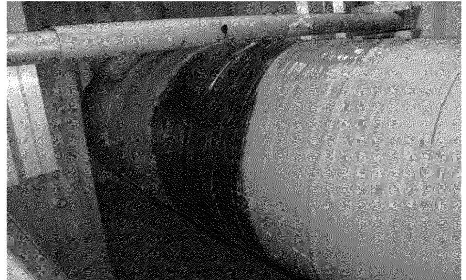
Overview of final coating condition US 3:00
