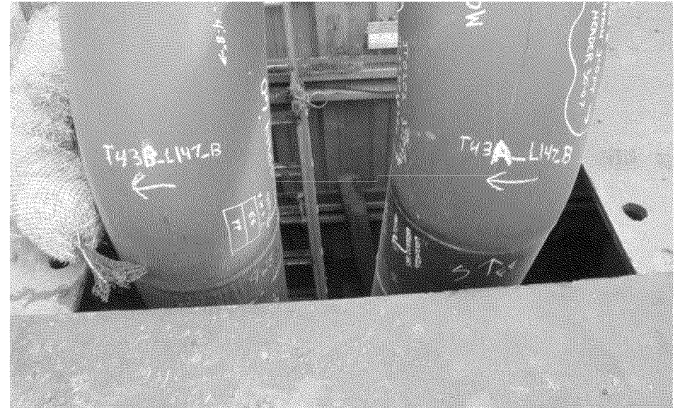
Closeup of T43A(US) & T43B(DS) in same excavation.
