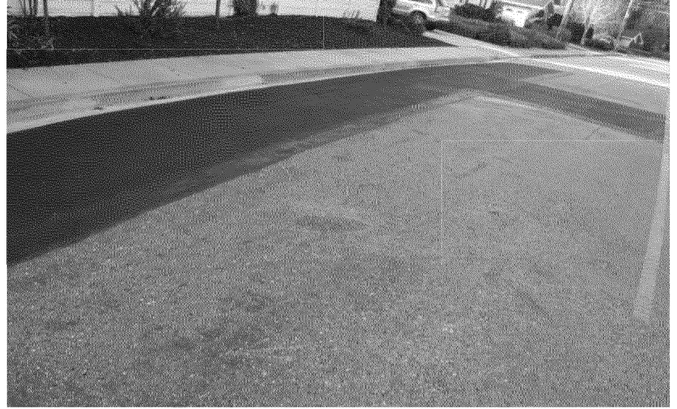
Overview of completed Cover, 9:00 view
