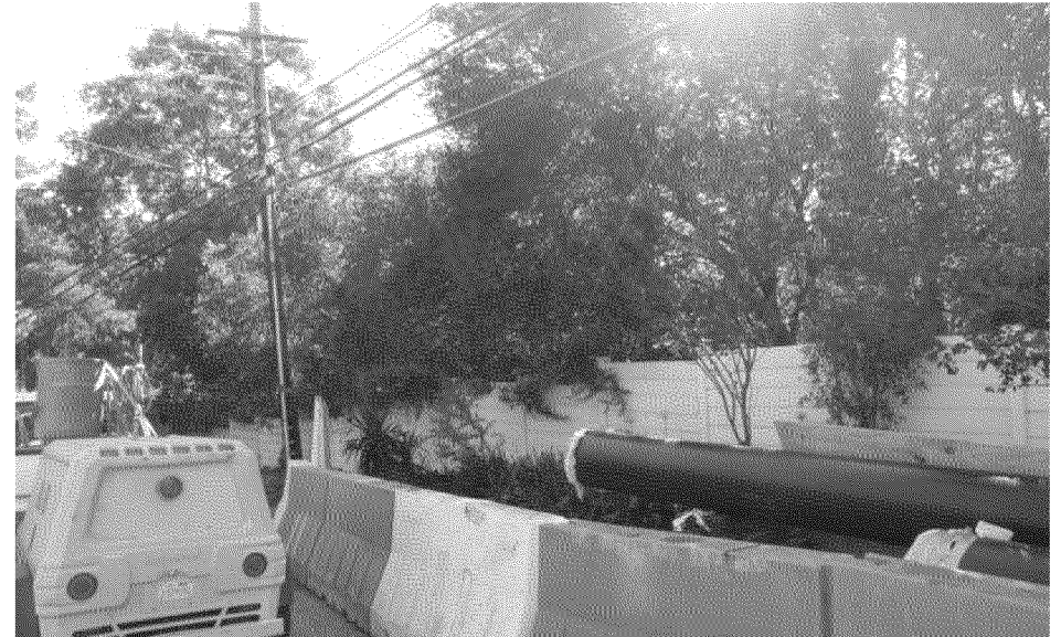
Typical surrounding topography
