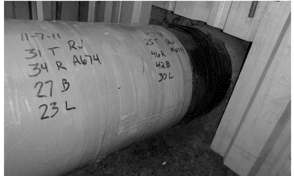
Overview of final coating condition US 3:00
