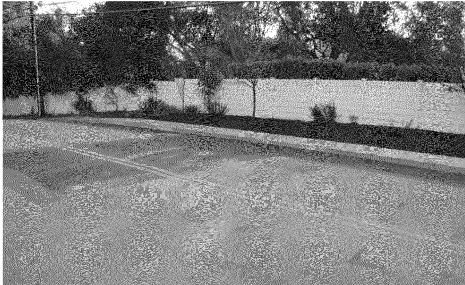
Overview of completed Cover looking upstream
