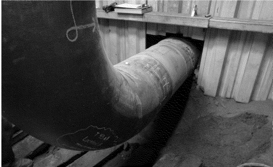
Overview of MPI layout -1ft to 2ft, 9:00 position
