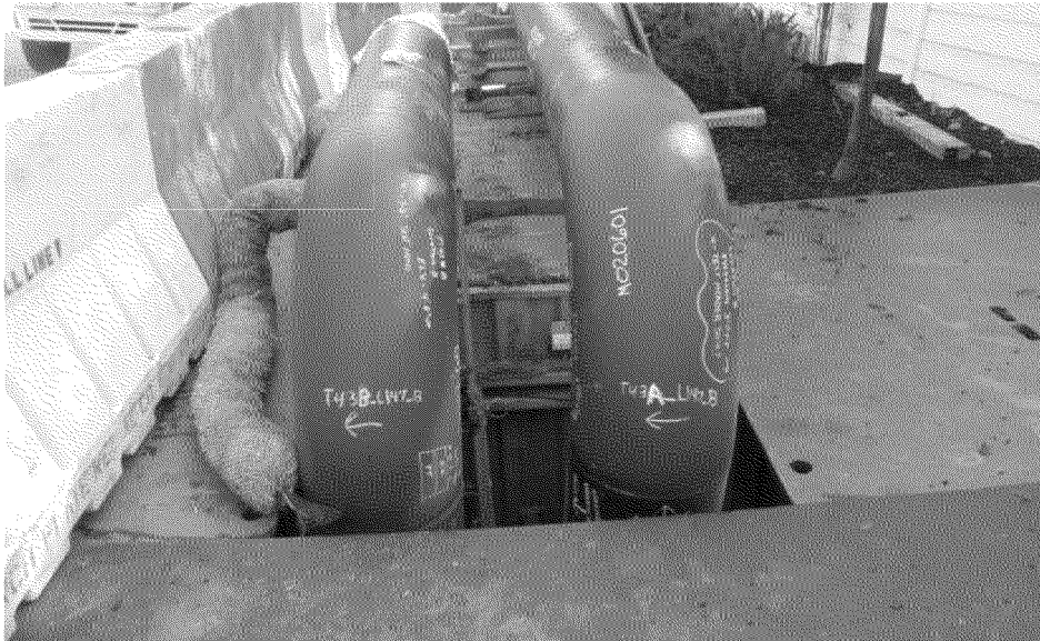
Overview of T43A(US) & T43B(DS) in same excavation.
