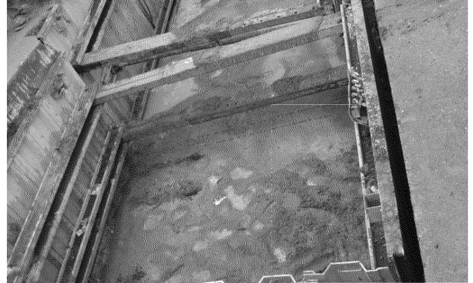
Overview of completed Slurry
