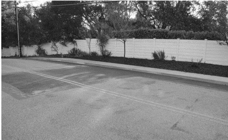
Overview of completed Cover looking upstream
