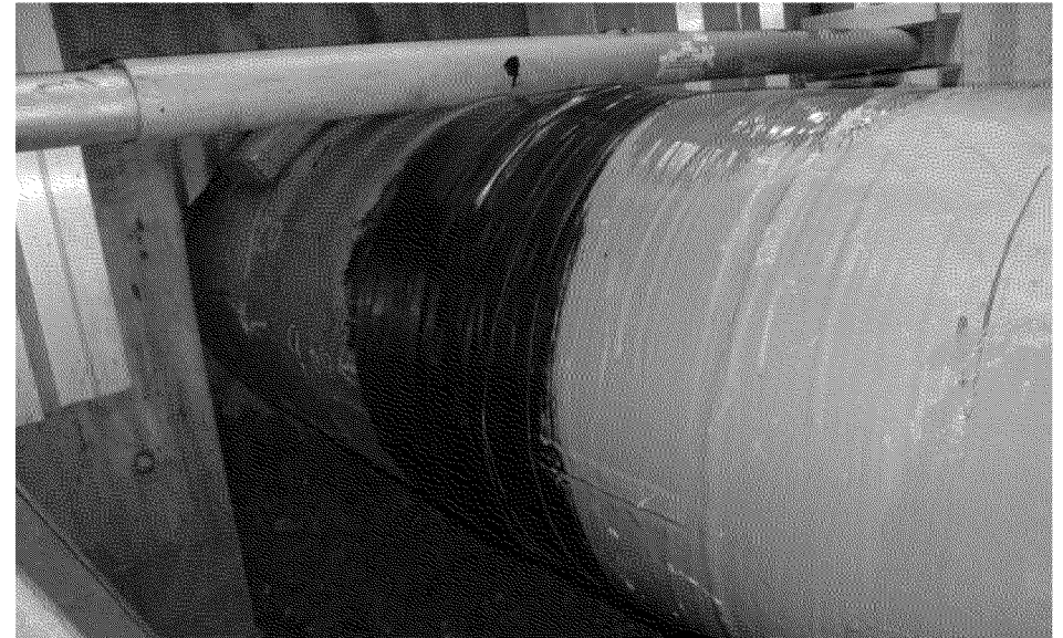
Overview of final coating condition US 3:00
