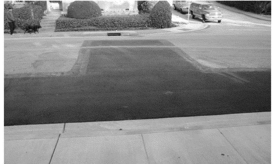
Overview of completed Cover looking downstream
