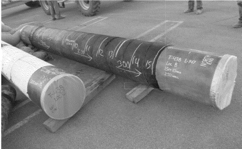
Removed pipe section coating assesment 3:00
