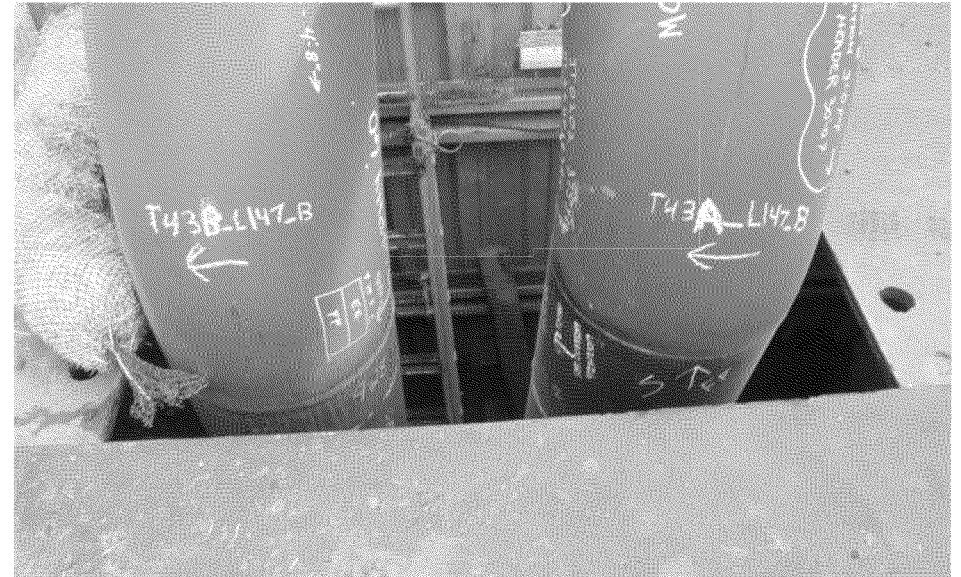
Closeup of T43A(US) & T43B(DS) in same excavation.
