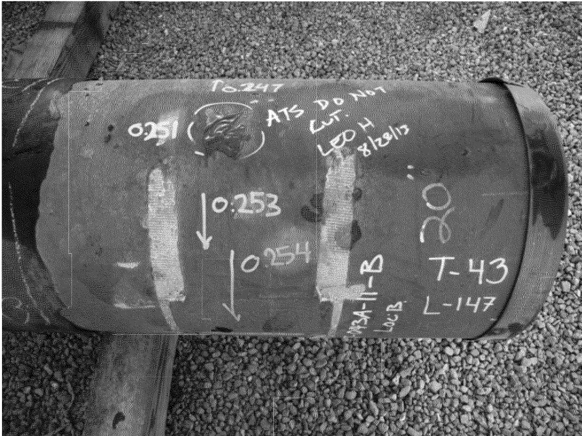
Downstream end of spool
