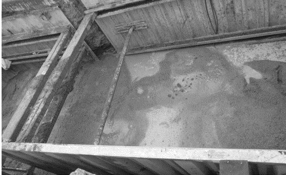
Overview of completed Slurry
