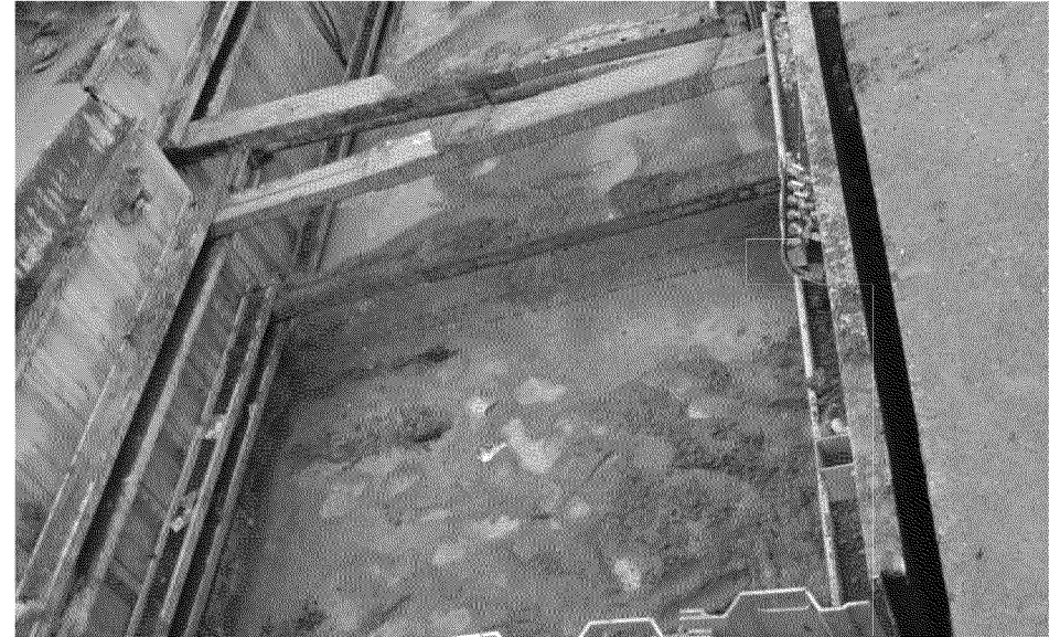
Overview of completed Slurry
