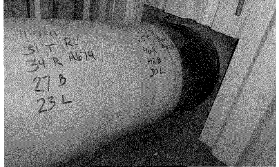
Overview of final coating condition US 3:00
