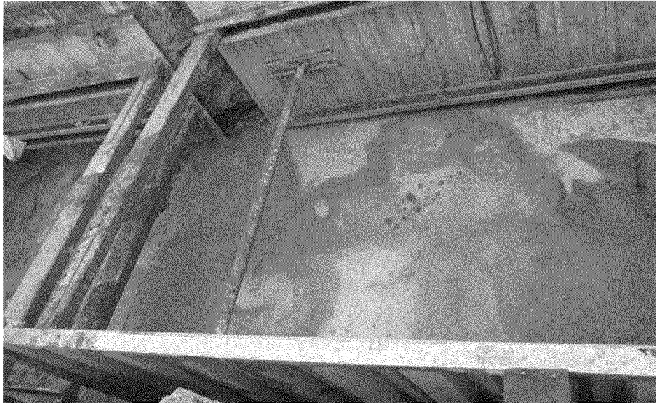
Overview of completed Slurry
