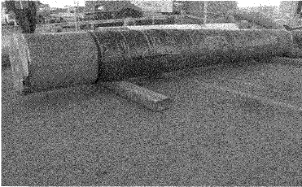
Removed pipe section coating assesment 9:00
