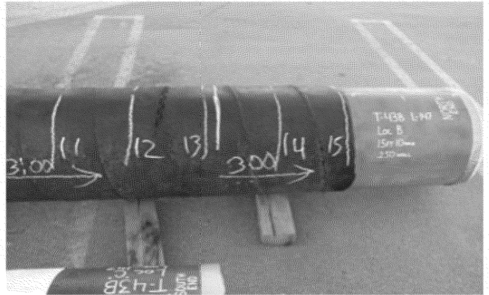
Overview of coating condition 3:00 position
