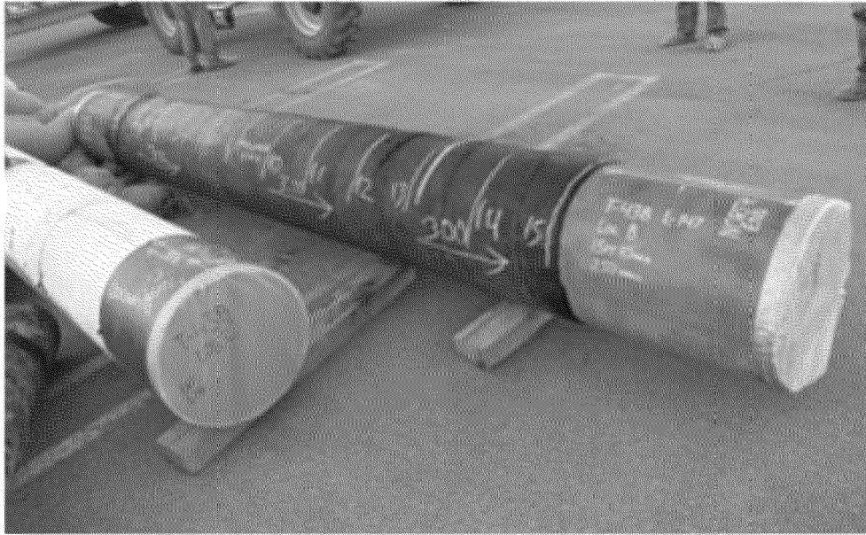
Removed pipe section coating assesment 3:00
