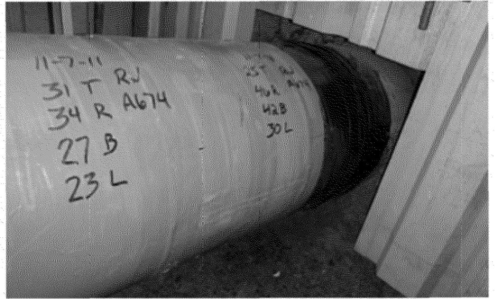
Overview of final coating condition US 300
