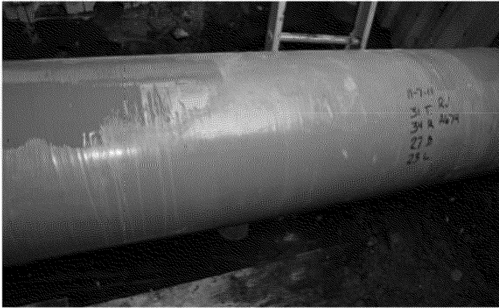
Overview of final coating condition 3:00
