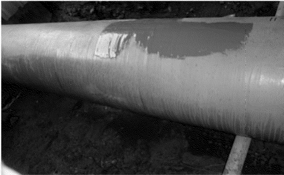
Overview of final coating condition 3:00
