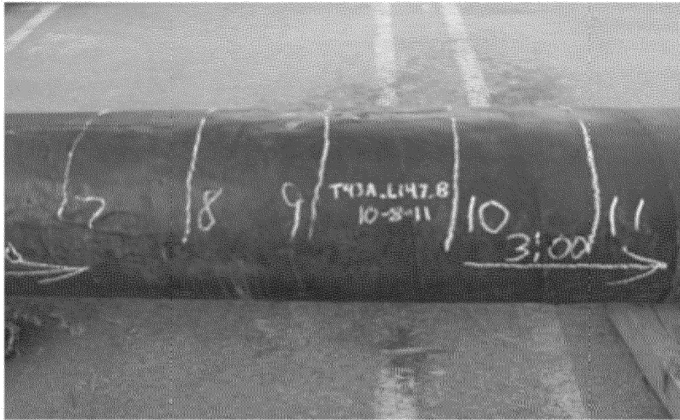
Overview of coating condition 300 position
