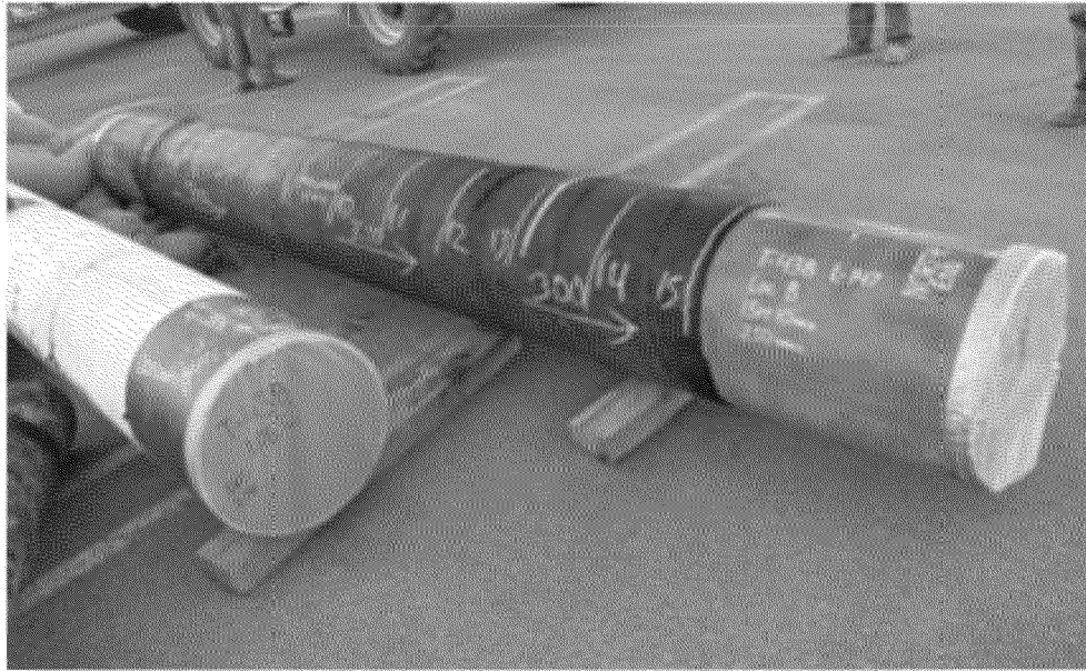
Removed pipe section coating assesment 3:00
