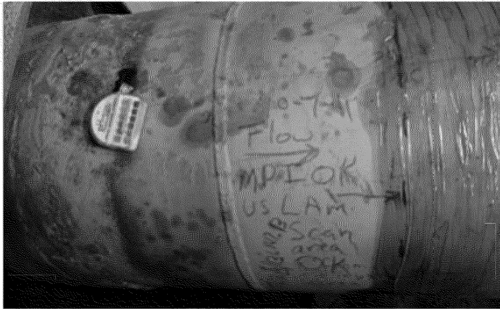
Overview of pipe Ph.
