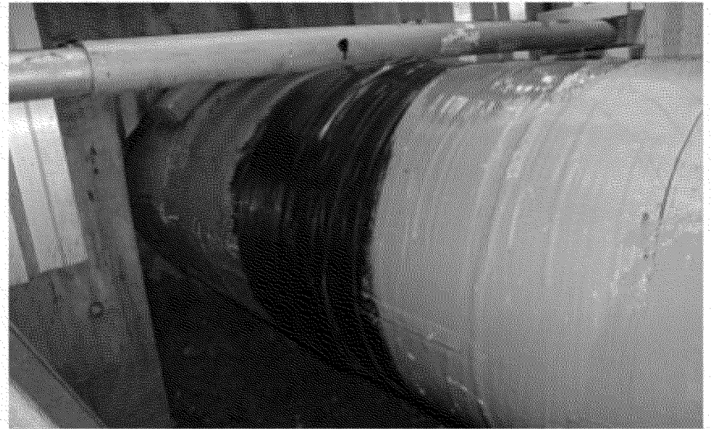
Overview of final coating condition US 3:00
