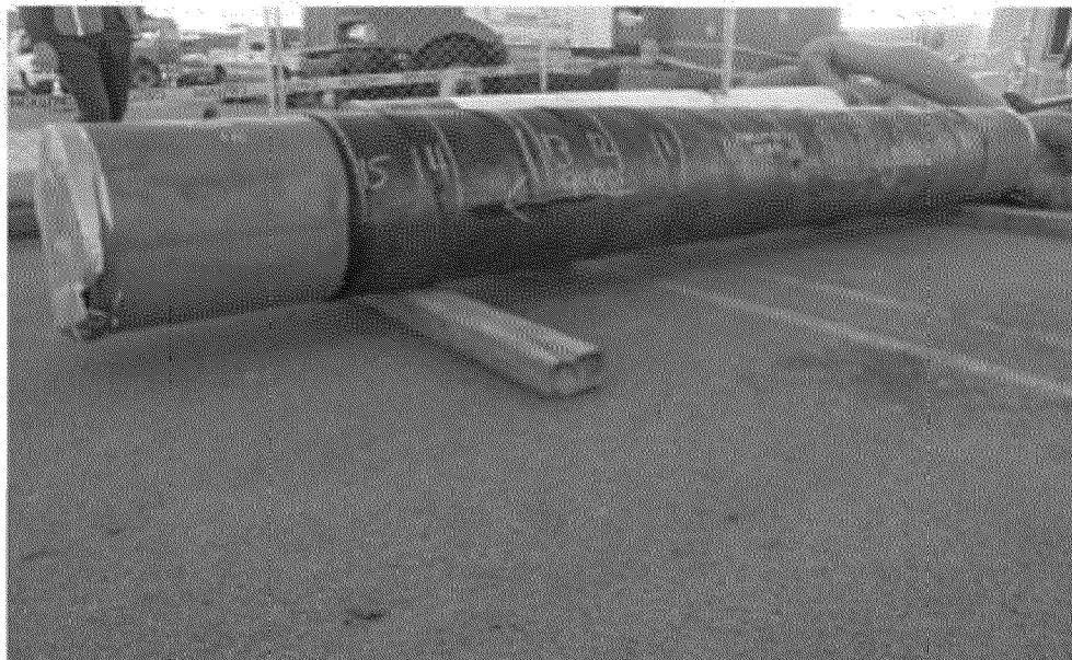
Removed pipe section coating assesment 9:00
