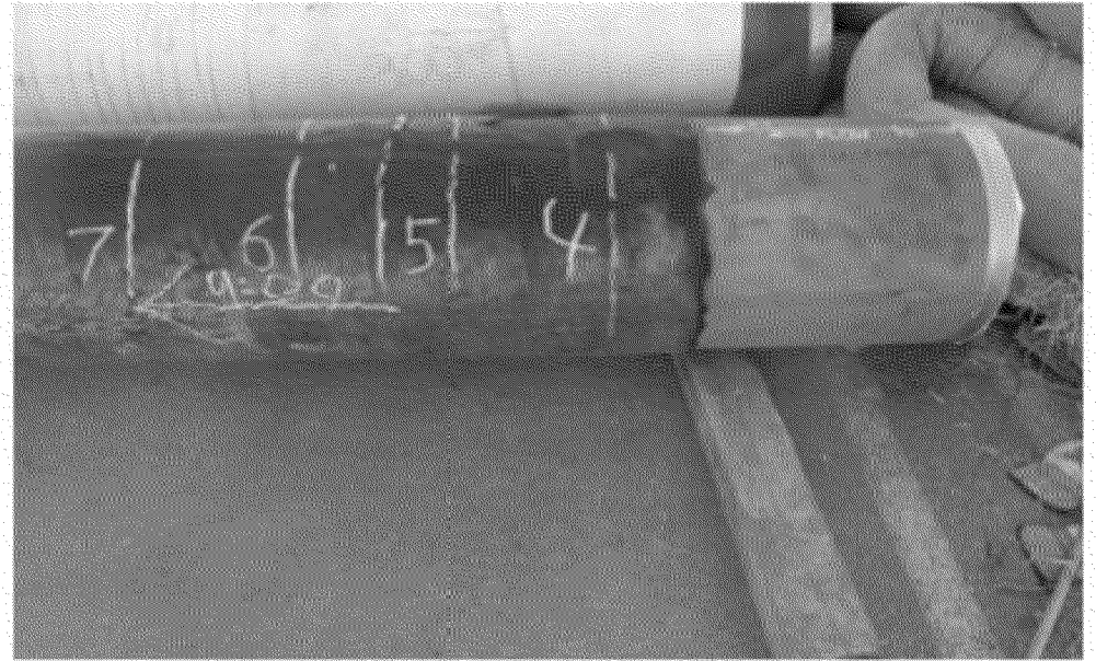
Overview of coating condition 9:00 position
