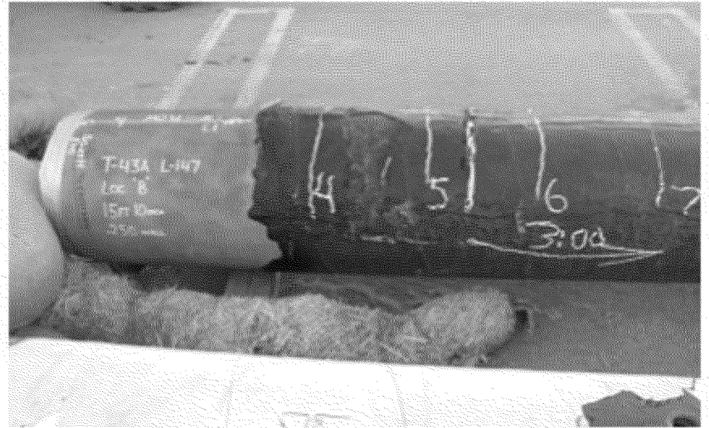
Overview of coating condition 3:00 position
