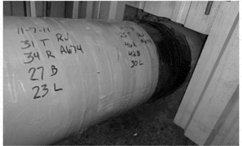
Overview of final coating condition US 300
