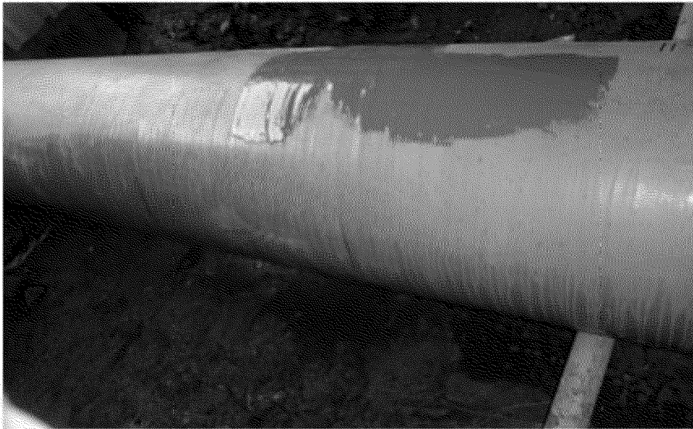
Overview of final coating condition 3:00
