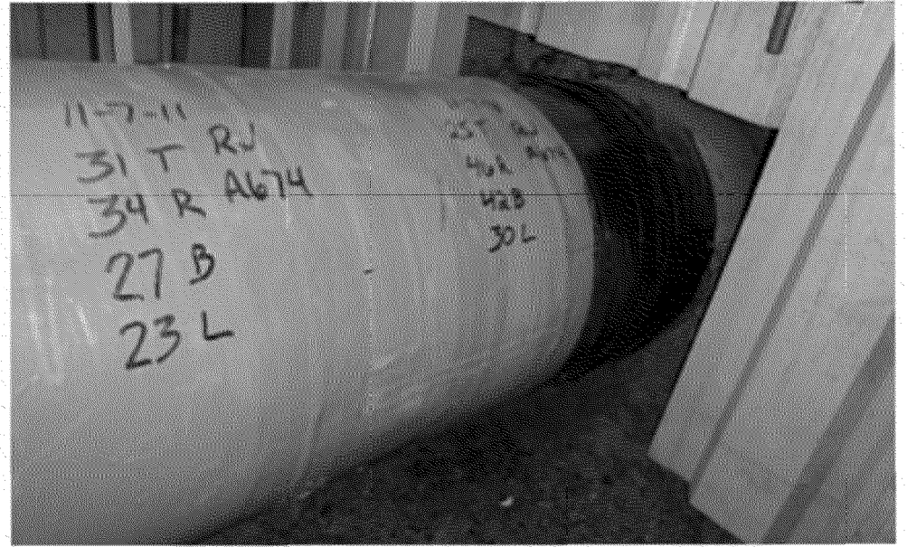
Overview of final coating condition US 300
