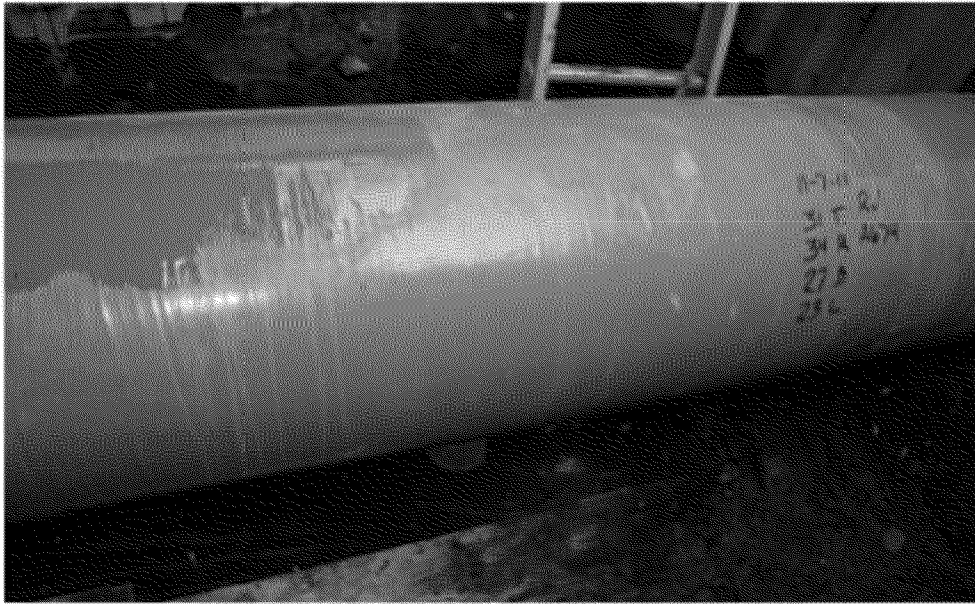
Overview of final coating condition 3:00
