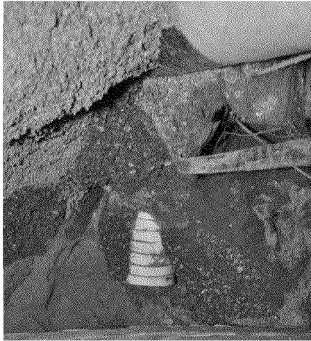
3" and 4" gas mains and sewer line
