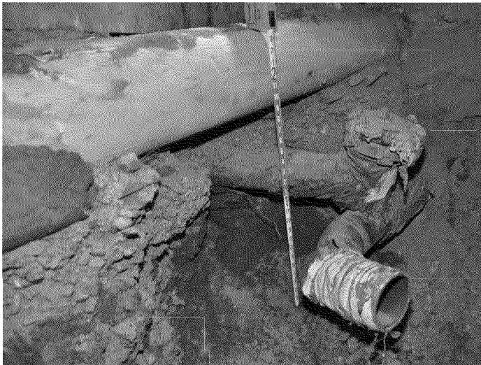
3" and 4" gas mains and sewer line
