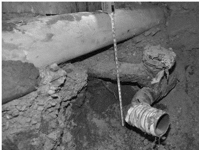
3" and 4" gas mains and sewer line
