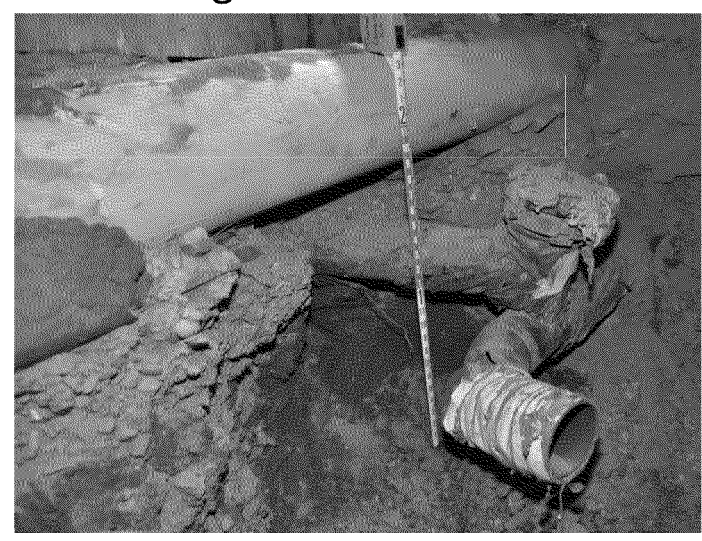
3" and 4" gas mains and sewer line
