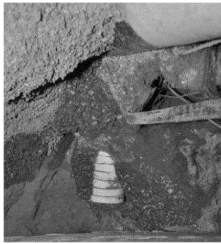
3" and 4" gas mains and sewer line
