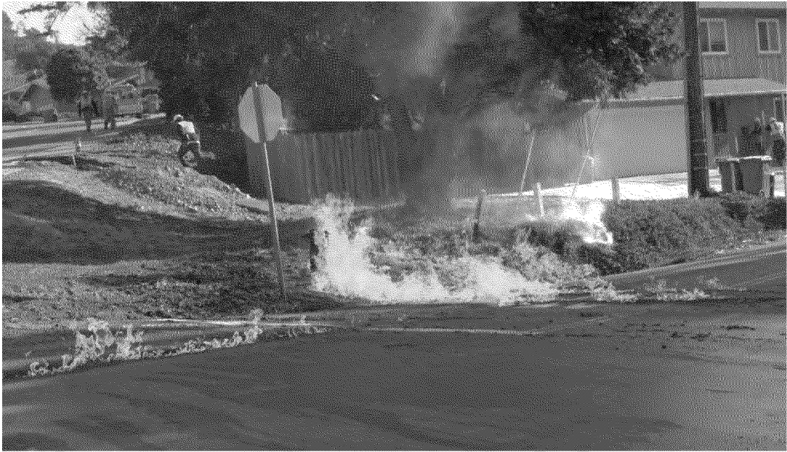
Figure 2. Image of the fire resulting from gas release. Source: PG&E
