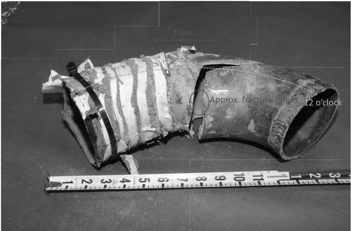
Figure 15. Image of fractured elbow.
