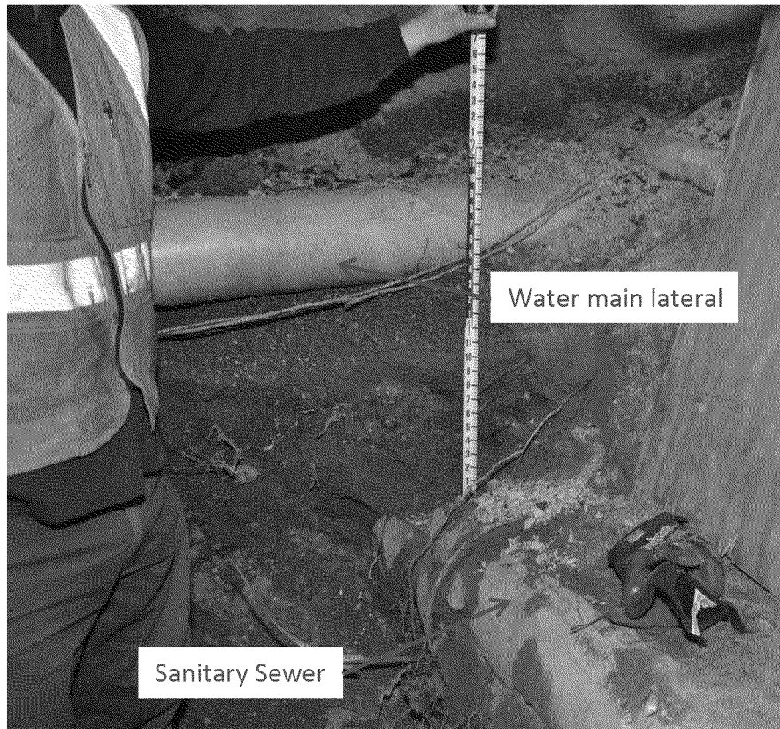
Figure 13. Water main lateral and sanitary sewer.
