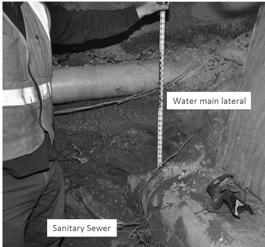
Figure 13. Water main lateral and sanitary sewer.
