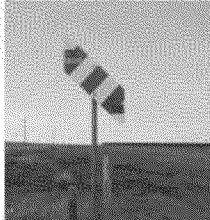
Markers like the ones above identify the general location of PG&E pipelines.
