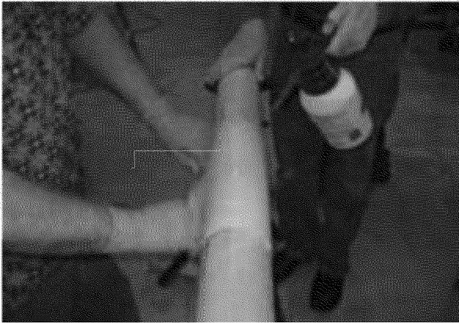
Composite repair trial on polyethylene pipe.
