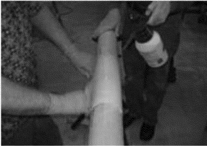
Composite repair trial on polyethylene pipe.
