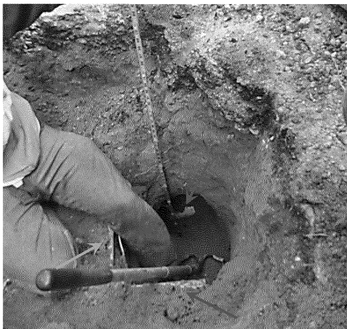
Figure 45. Excavation to expose sewer lateral at subject residence in the vicinity of gas service tee. Yellow arrow indicates gas main along Redacted Redacted Redacted. Red arrow indicates gas service line. Green arrow indicates sewer lateral. Photograph by Exponent on March 21, 2014.
