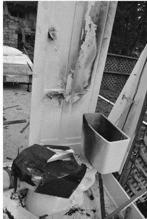
Figure 14. Bathroom toilet. Photograph by Exponent on March 6, 2014.
