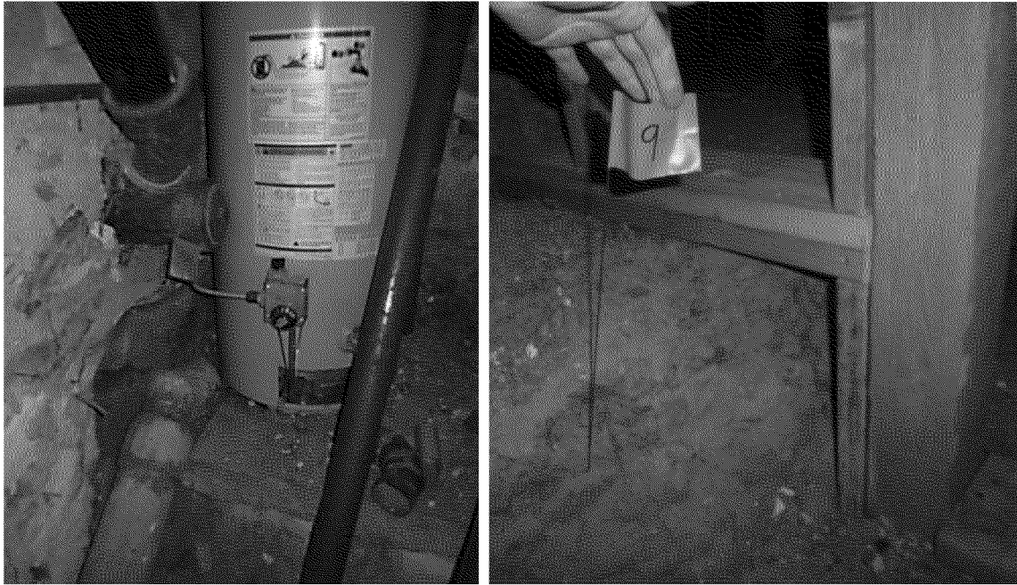
Figure 56. Example monitoring points at the residence's basement. Monitoring point #8 (left) by the cleanout next to water heater. Monitoring point #9 (right) near center of basement, over soil. Photographs by Exponent on March 21, 2014.
