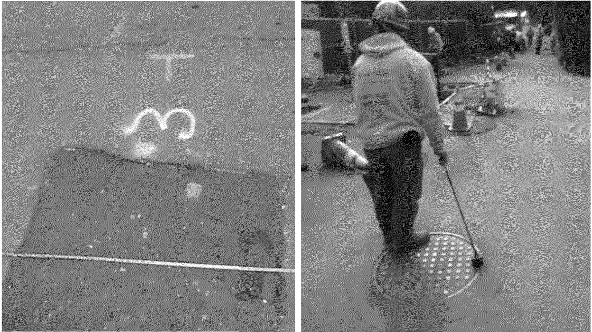
Figure 55. Example monitoring points outside of residence. Monitoring point #3 (left) near excavation performed by PG&E at gas service tee for residence. Monitoring point #19 (right) at sewer manhole near the [Redacted] [Redacted] Photographs by Exponent on March 21, 2014.
