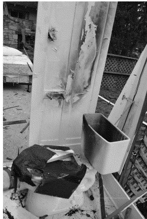
Figure 14. Bathroom toilet. Photograph by Exponent on March 6, 2014.
