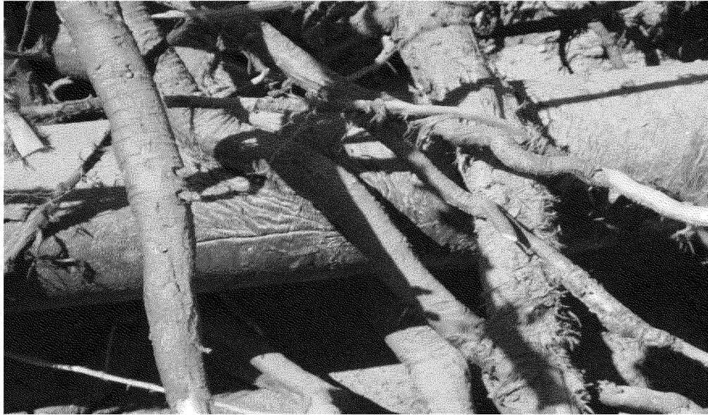
Figure 3. RWVIM-107-13 (Weber Lane) (CTE coating damage)
