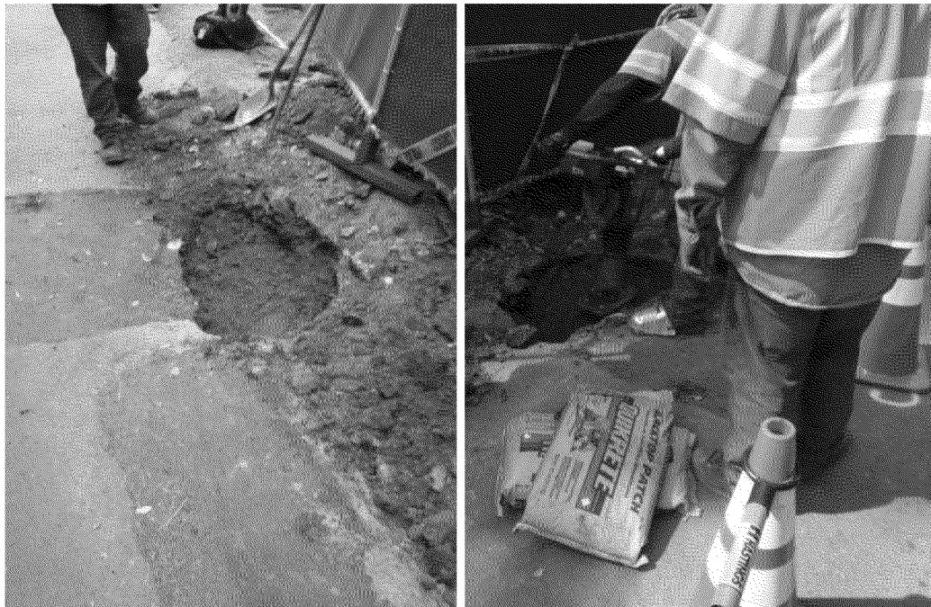
Figure 58. Excavation (left) and re-compaction (right) near gas service tee. Photographs by Exponent on March 21, 2014.
