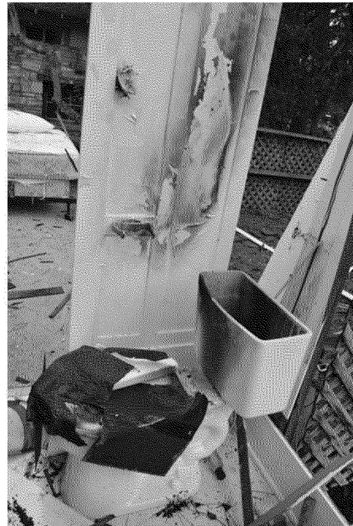
Figure 14. Bathroom toilet. Photograph by Exponent on March 6, 2014.
