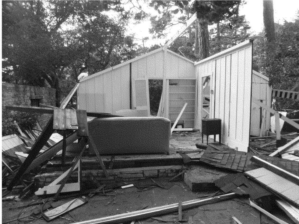
Figure 9. Incident house looking West from the entryway. Photograph by Exponent on March 4, 2014.
