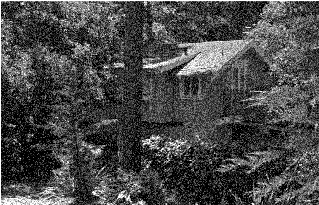
Figure 7. Pre-incident photo of the house, looking southeast from [Redacted]. Source: Google Maps street view.
