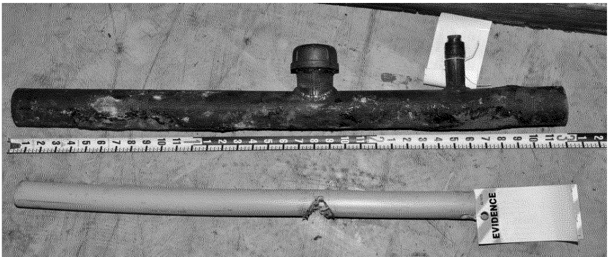
Figure 27. Portion of the gas main along [Redacted] Steel pipe (top) with welded fittings and plastic pipe insert. Photograph by Exponent on March 10, 2014.
