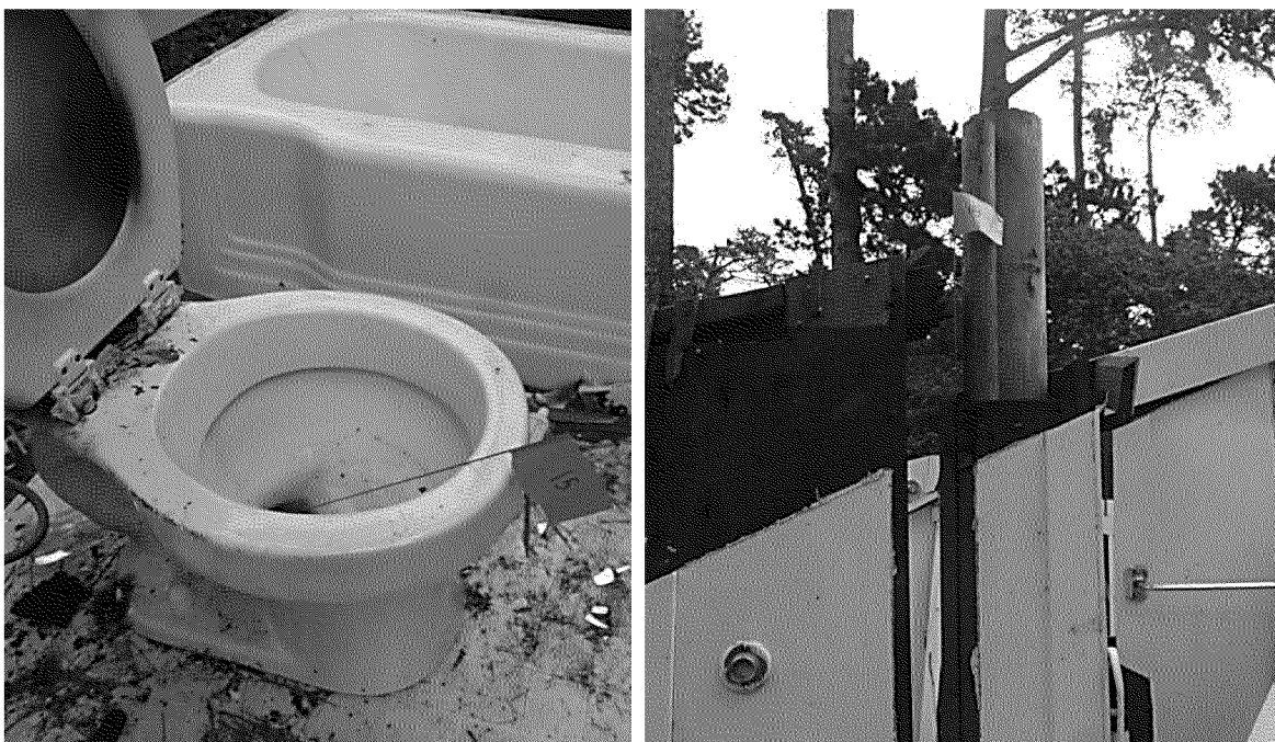
Figure 57. Example monitoring points at the residence's first floor. Monitoring point #15 (left) at the toilet. Monitoring point #18 (right) at bathroom vents. Photographs by Exponent on March 21, 2014.
