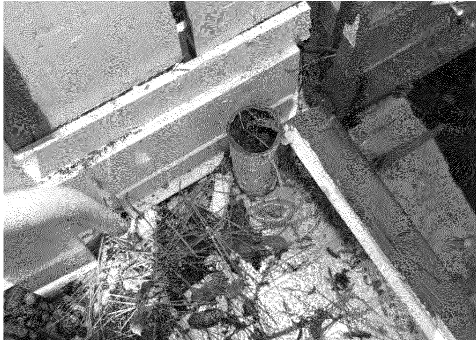
Figure 18. Sewer vent pipe (broken off) in the laundry room. Vent pipe likely broken off during the explosion. Photograph by Exponent on March 7, 2014.
