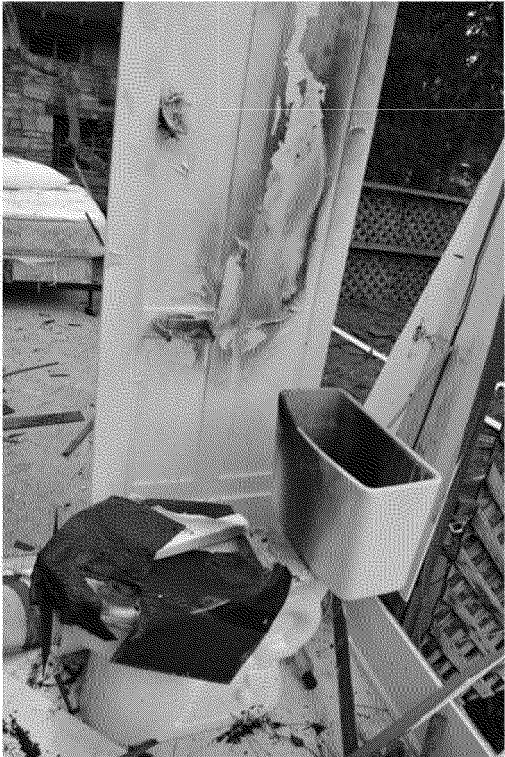
Figure 14. Bathroom toilet. Photograph by Exponent on March 6, 2014.
