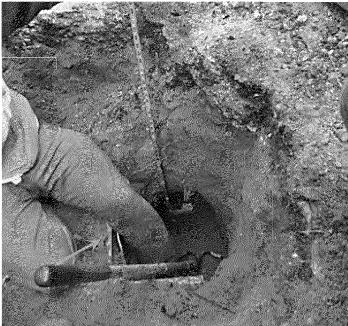
Figure 45. Excavation to expose sewer lateral at subject residence in the vicinity of gas service tee. Yellow arrow indicates gas main along [Redacted] [Redacted] Red arrow indicates gas service line. Green arrow indicates sewer lateral. Photograph by Exponent on March 21, 2014.
