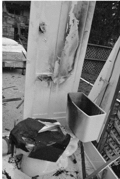
Figure 14. Bathroom toilet. Photograph by Exponent on March 6, 2014.
