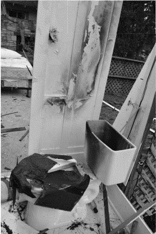
Figure 14. Bathroom toilet. Photograph by Exponent on March 6, 2014.
