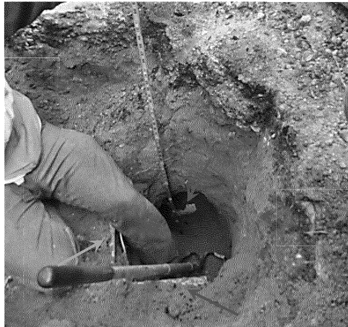
Figure 45. Excavation to expose sewer lateral at subject residence in the vicinity of gas service tee. Yellow arrow indicates gas main along 3 rd Avenue. Red arrow indicates gas service line. Green arrow indicates sewer lateral. Photograph by Exponent on March 21, 2014.
