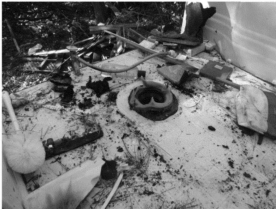
Figure 39. Toilet removed to allow for insertion of sewer push camera. Photograph by Exponent on March 11, 2014.
