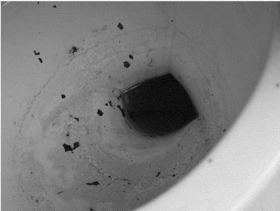
Figure 50. Low water level in the bathroom toilet bowl three days after explosion. Photograph by Exponent on March 6, 2014.
