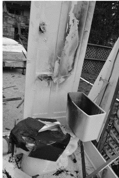
Figure 14. Bathroom toilet. Photograph by Exponent on March 6, 2014.
