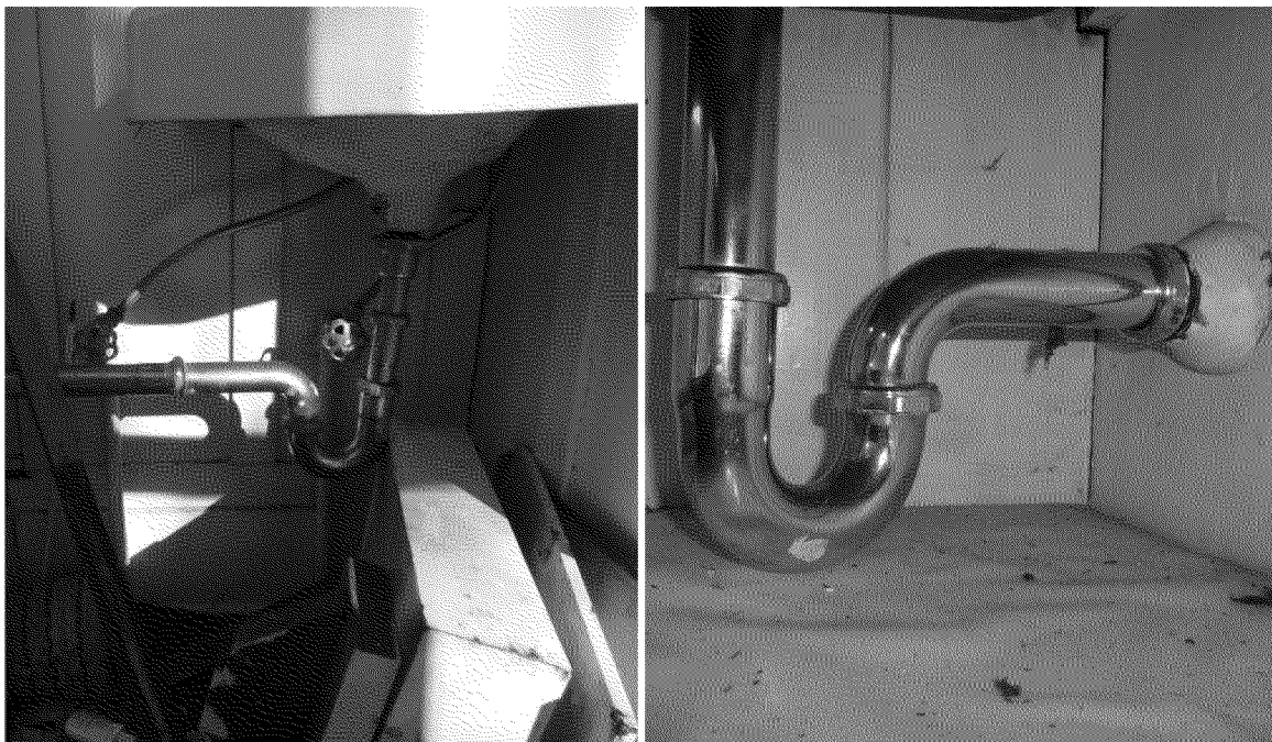
Figure 48. Plumbing traps at bathroom sink (left) and kitchen sink (right). Photographs by Exponent on March 11, 2014.
