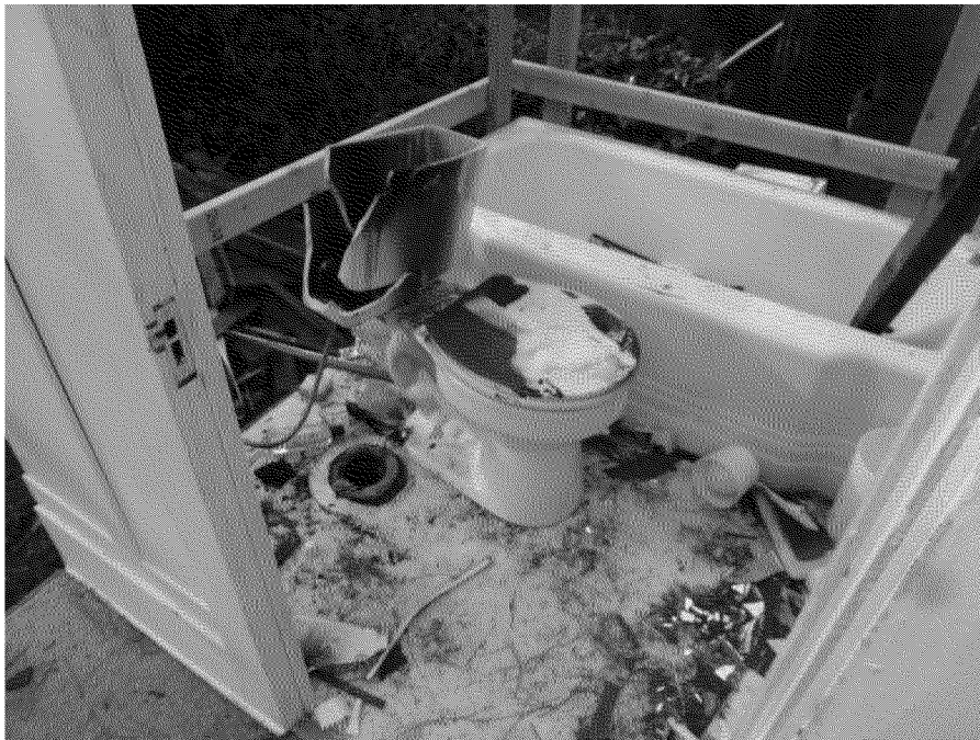
Figure 59. Monitoring point #15 after removal of the toilet. Photograph by Exponent on March 21, 2014.
