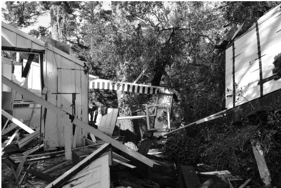
Figure 10. Incident house looking West into the laundry room. Roof section on right side of picture. Photograph by Exponent on March 4, 2014.
