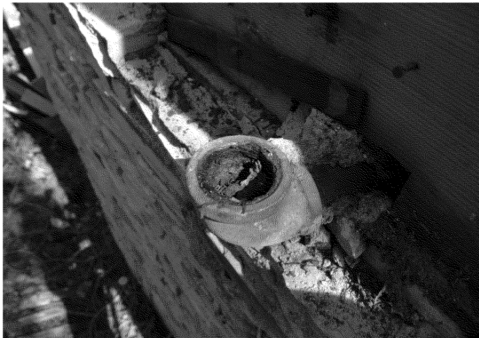
Figure 19. Vent pipe (broken off) in the bathroom. Photograph by Exponent on March 7, 2014.
