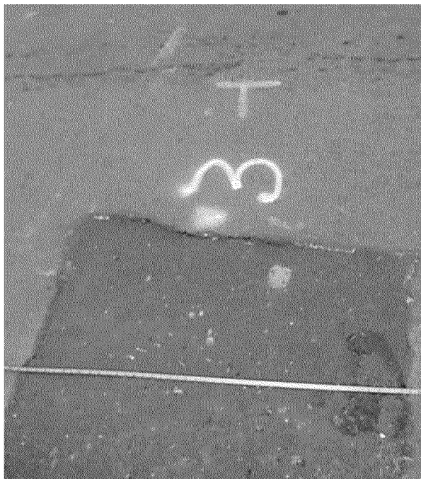
Figure 55. Example monitoring points outside of residence. Monitoring point #3 (left) near excavation performed by PG&E at gas service tee for residence. Monitoring point #19 (right) at sewer manhole near the intersection of Red Redacted Photographs by Exponent on March 21, 2014.
