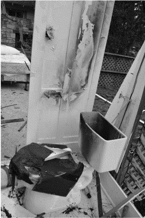
Figure 14. Bathroom toilet. Photograph by Exponent on March 6, 2014.
