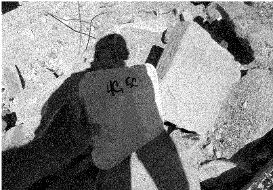
Sample 5C 12 Inch Tile Grout - Boiler 4
