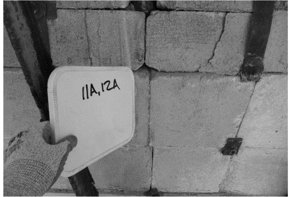
Sample 11A 12 Inch Tile - Boiler 2
