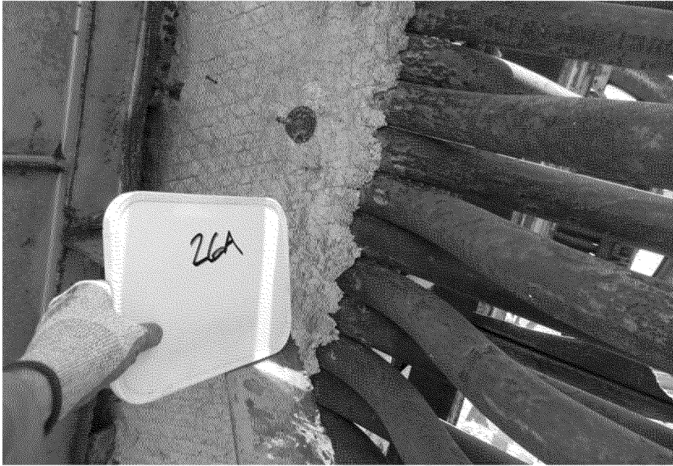
Sample 26A Refractory - Boiler 1
