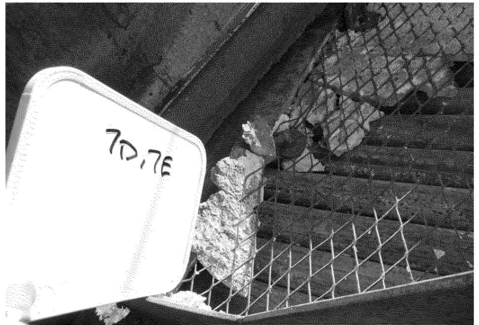
Sample 7E Refractory - Boiler 4
