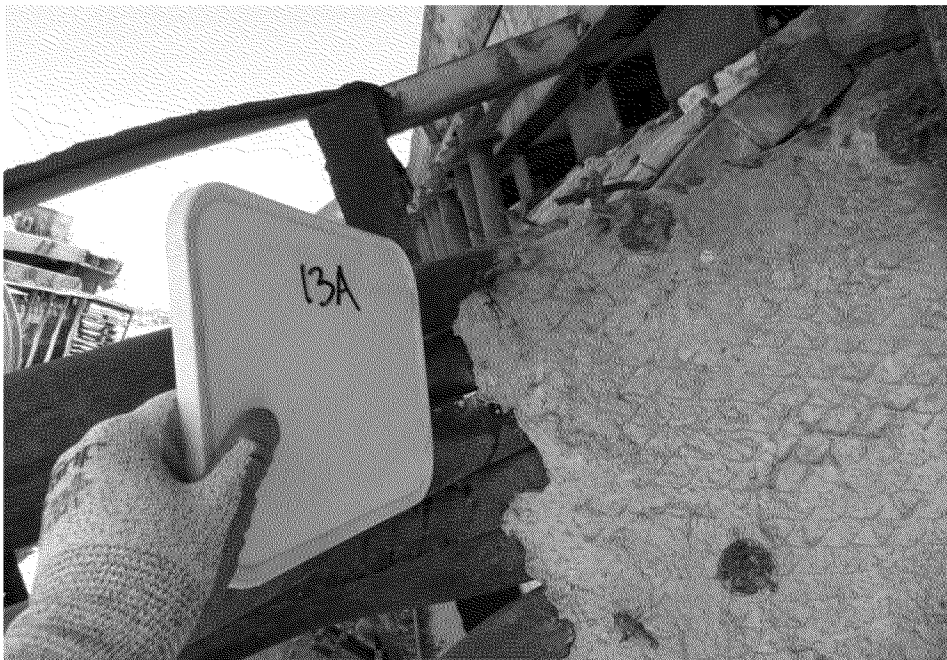
Sample 13A Refractory - Boiler 2
