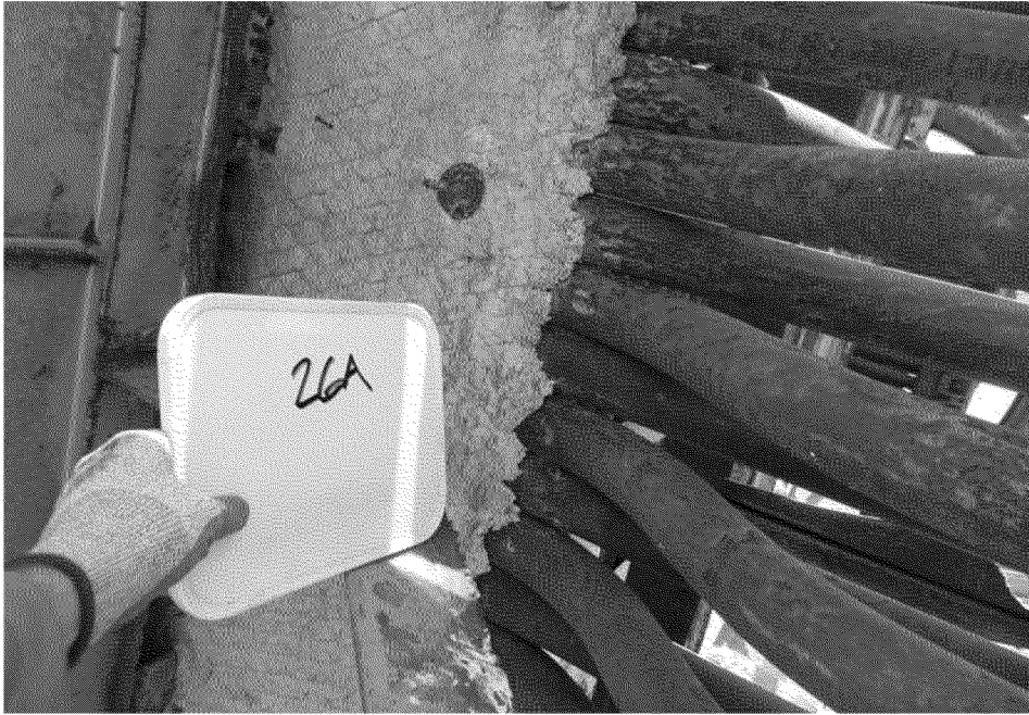
Sample 26A Refractory - Boiler 1
