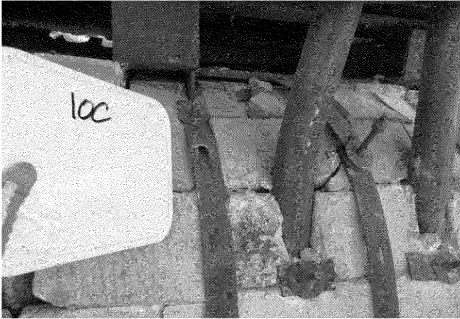
Sample 10C Misc. Tile Grout - Boiler 2
