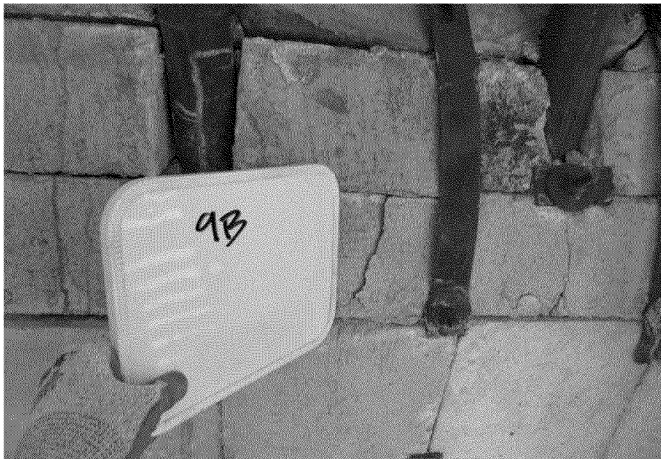
Sample 9B Misc. Tile - Boiler 2
