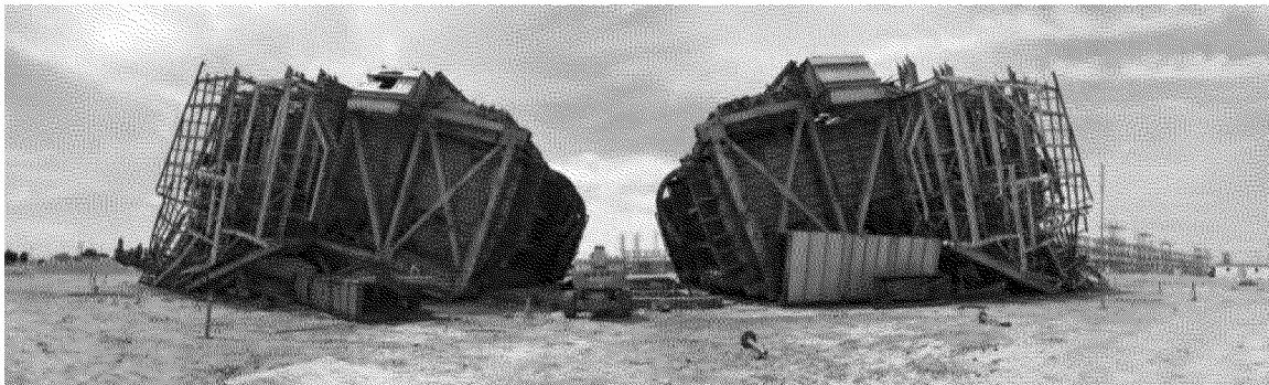
Felled Boiler Structures (View Looking South)
