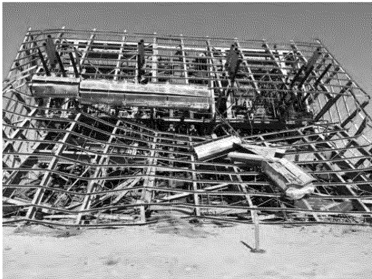
Former Top of Boiler Structures (East End, View Looking West)
