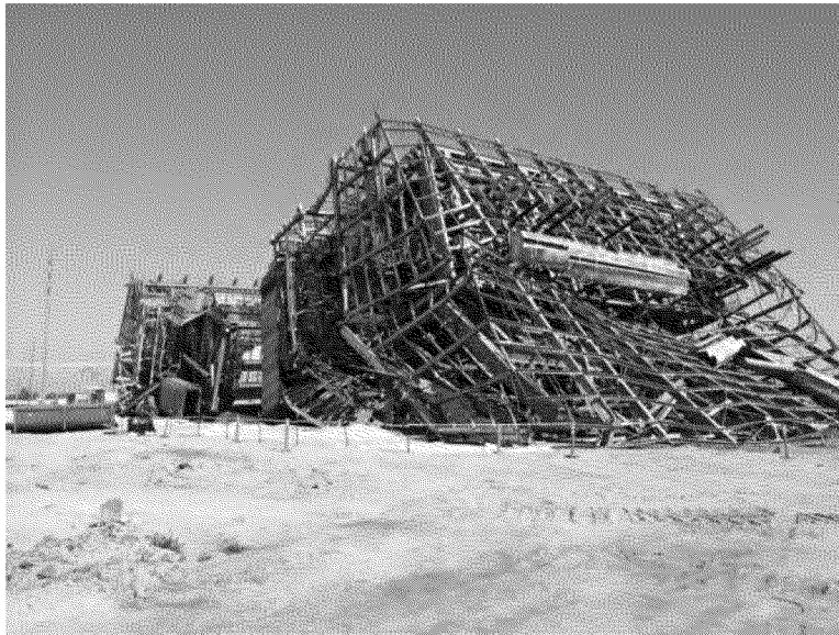
Northwest Corner of Boiler Structures (View Looking SW)
