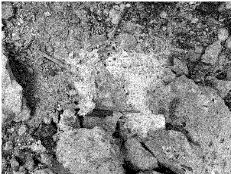
TSI Debris Between Boiler Structures (Closeup View)
