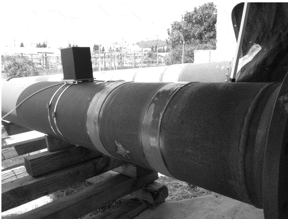
A data acquisition box sits atop a test pipe wrapped with sensors and covered with protective fiberglass (yellow bands) as part of new technology to remotely monitor pipeline health.
