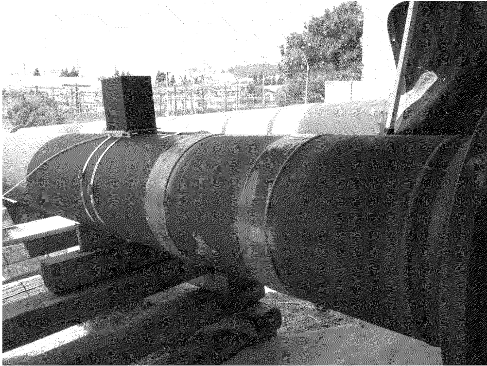
A data acquisition box sits atop a test pipe wrapped with sensors and covered with protective fiberglass (yellow bands) as part of new technology to remotely monitor pipeline health.
