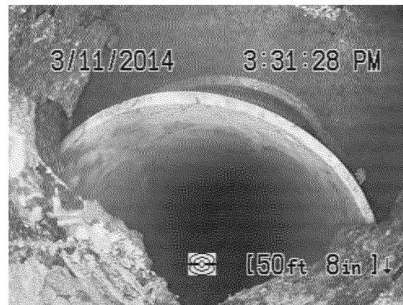
Figure 6. Offset joint 50 ft. from entry on property
