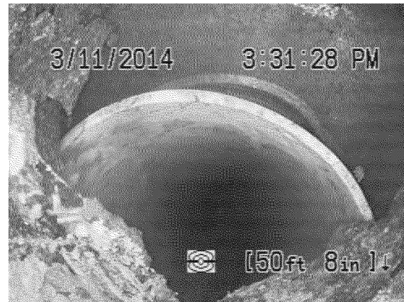
Figure 6. Offset joint 50 ft. from entry on property
