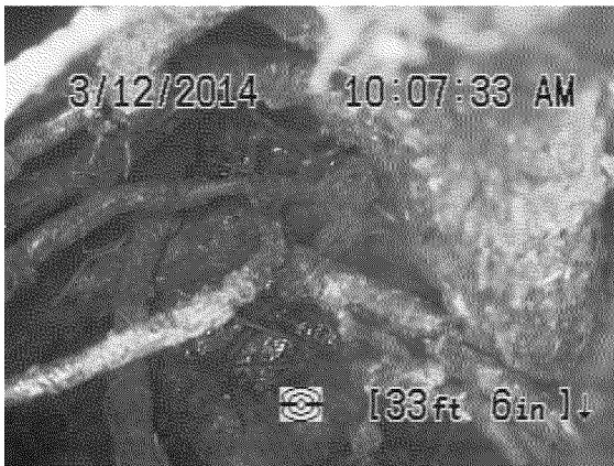
Figure 9. Lateral blocked by roots
