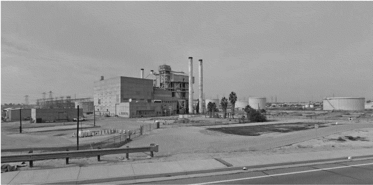
Figure 3: Kern Power Plant as seen from Coffee Road. Source: Google Maps.
