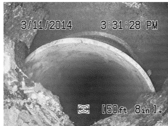
Figure 6. Offset joint 50 ft. from entry on property
